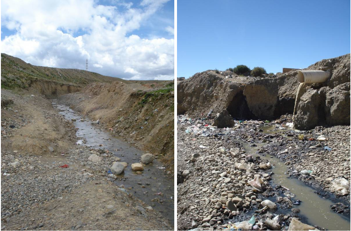
Figure 6. Photo on left shows RS-1 during January 2009 when there was water in the river. The photo on the right shows RS-1 during June, when the only water in the river was from raw sewage being discharged into the river.
