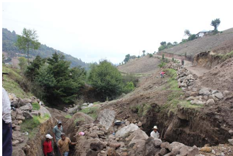
The community working in Ixcamal
