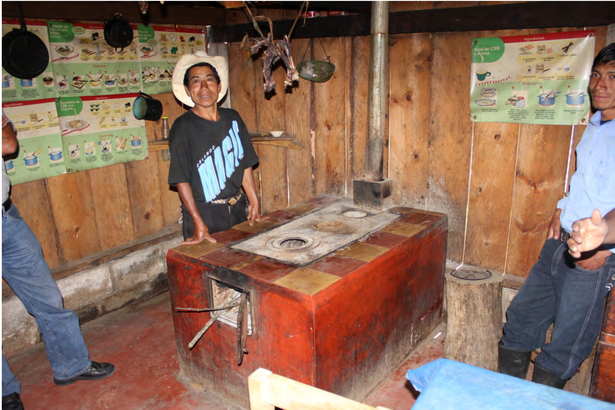
HFH Wood stoves, filters, and concrete floors
