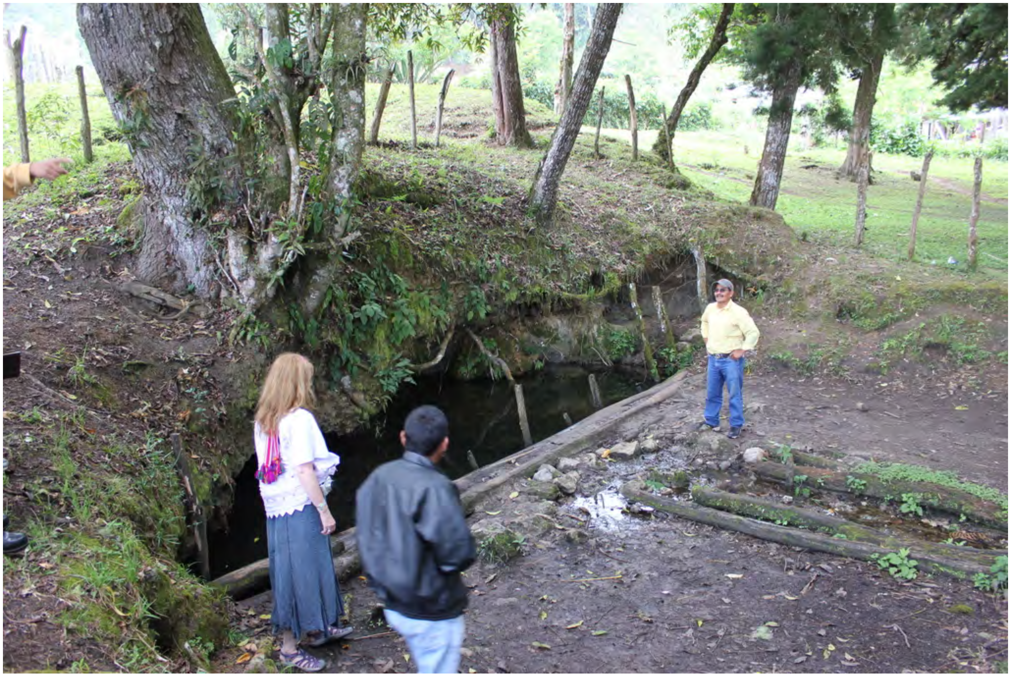
Village water source near year-round lake, in topographic low with high water table. Water collected from open, shallow wells
