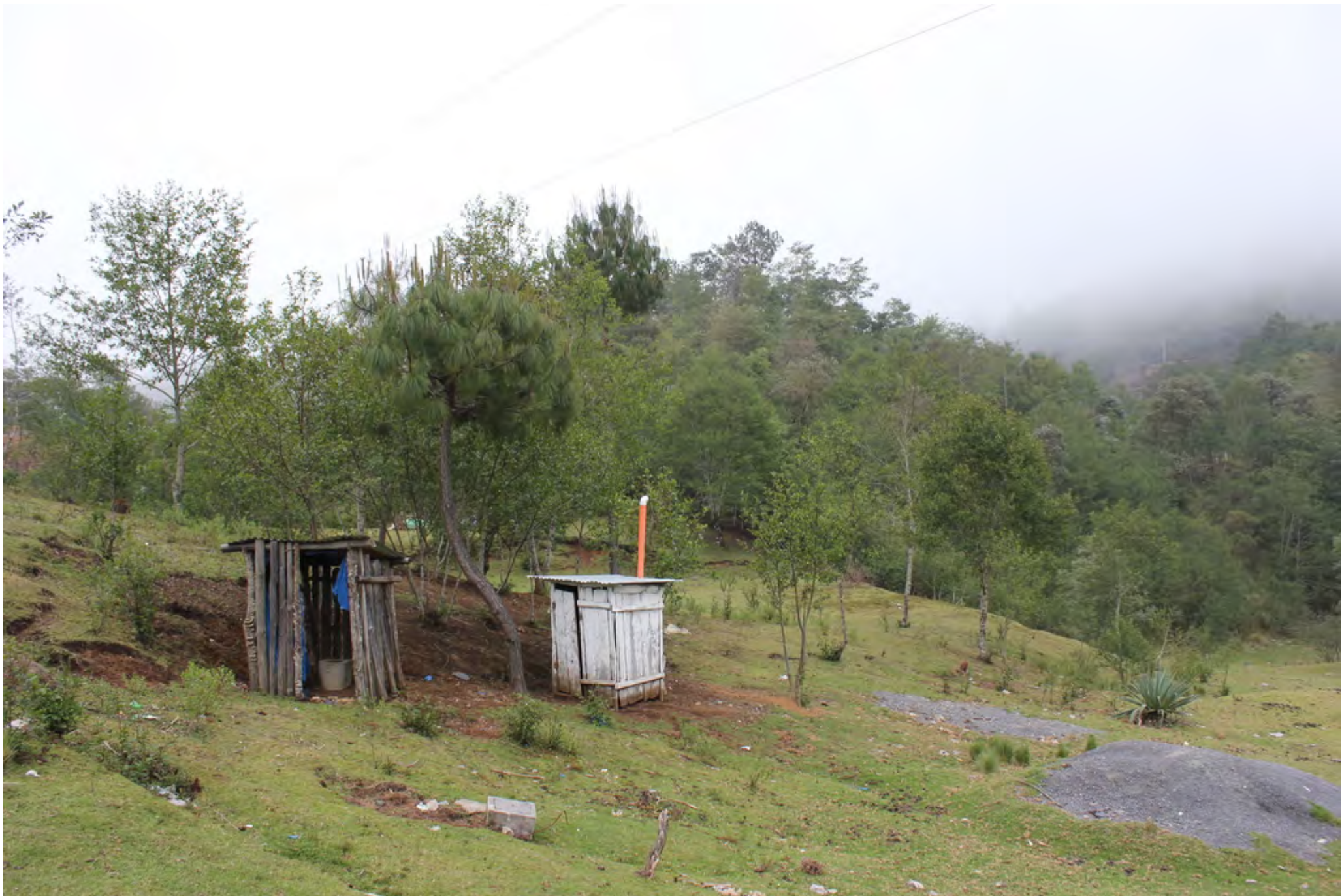
New Vented Latrine (right) near the replaced, unstable Latrine
