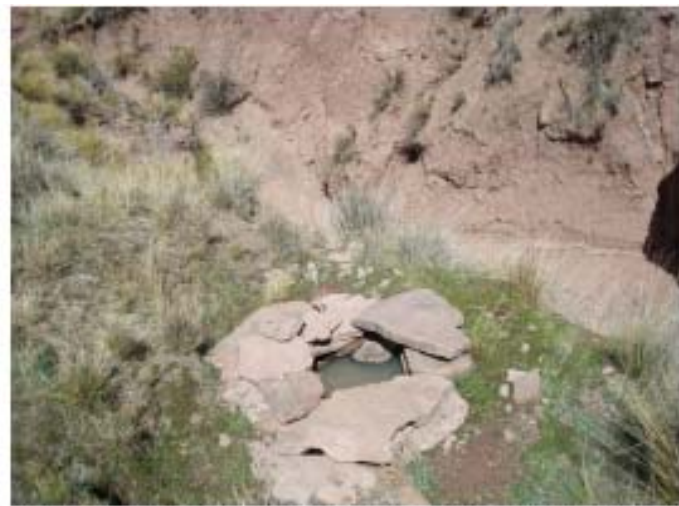
Typical community well, protected only with stones. The turbidity of the water can be observed.
