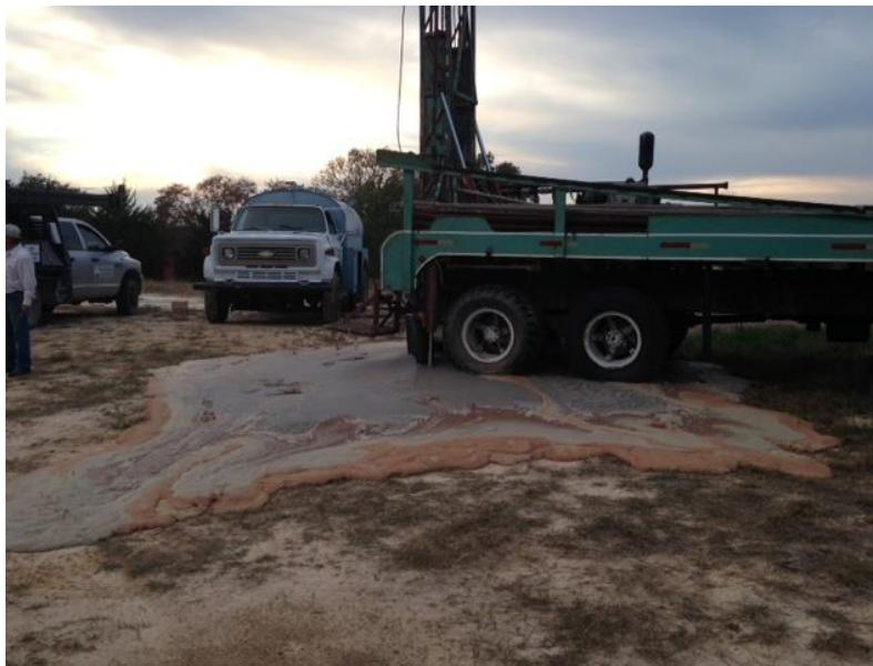
*During Braulio's visit to Texas and New Mexico in mid-October, he was introduced to foam drilling by Dale White, shown here. Dale explained the stops that would be needed if desired by Suma Jayma to retrofit their own drilling rig to be able to use compressed air/foaming agent in lieu of drilling mud with bentonite.*
