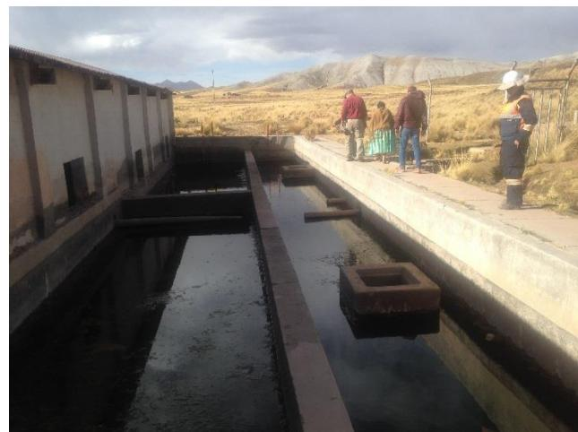
*Coro Coro Water Treatment Plant, built in 1976 and essentially abandoned since 1985, though water for mining activities still passes through the storage tanks. Surface water from a stream above bypasses this WTP and is fed to community of Coro Coro with no treatment. Tanks inside WTP building below.*
