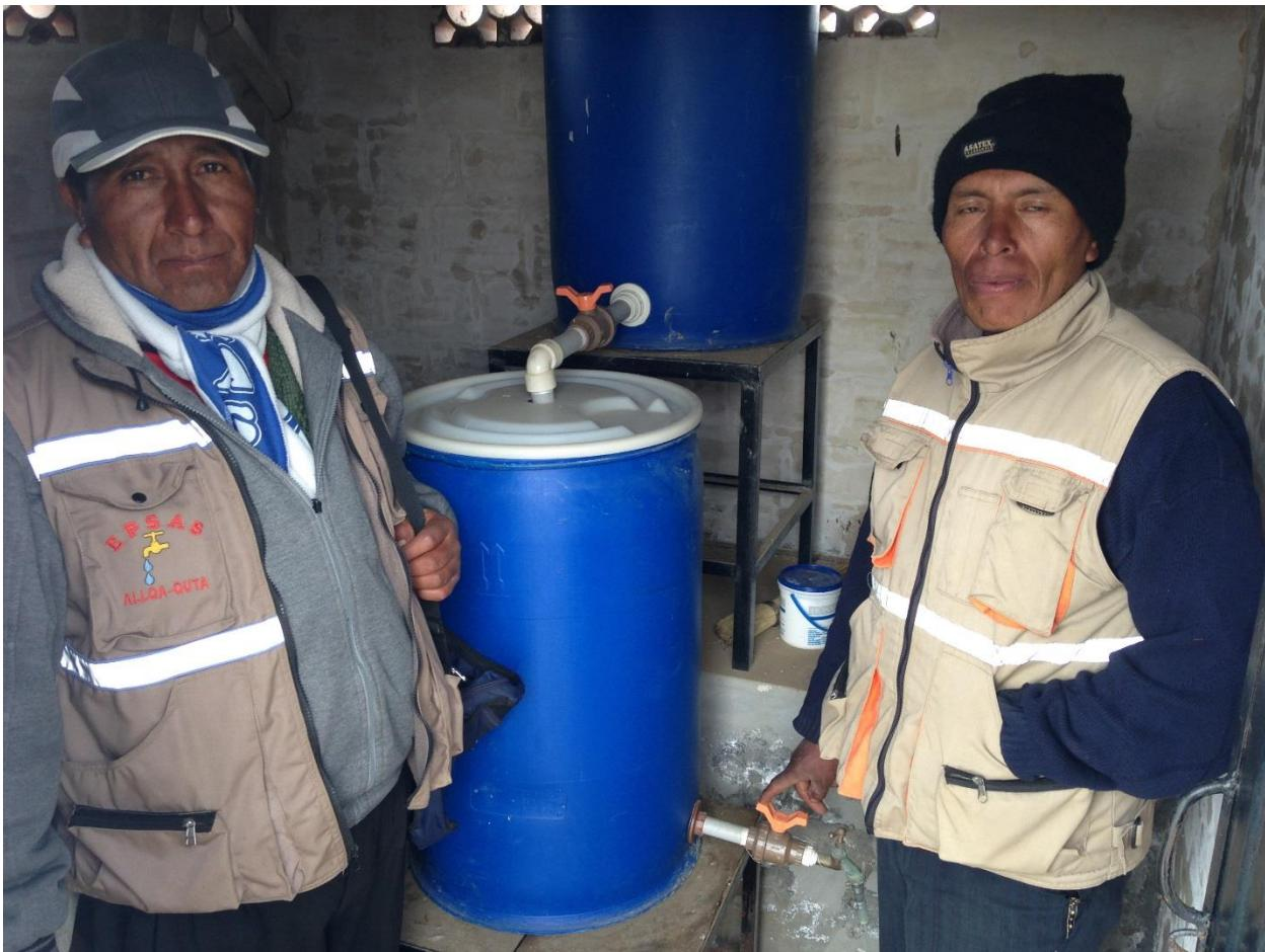
*Ensuring continuous and potable water for the eleven communities served by the drinking water association EPSAS "Allqa Quta" is the mission of its two operators, here seen keeping the chlorine solution drip into the 100 m<sup>3</sup> water supply tank operational.*
