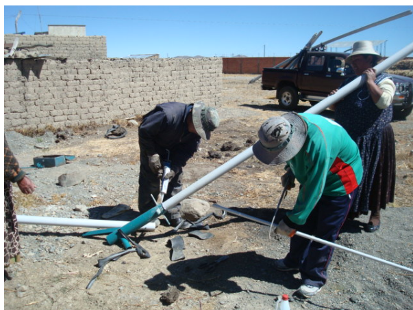
Jorge and Edgar of Suma Jayma complete construction of the pump mechanism to be installed
