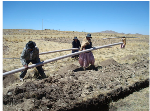
Families of Machacamarca helping with waterline installation
