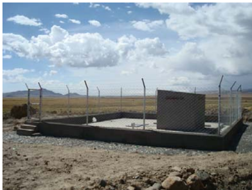
Underground water storage tank with chlorination building on top at Machacamarca
