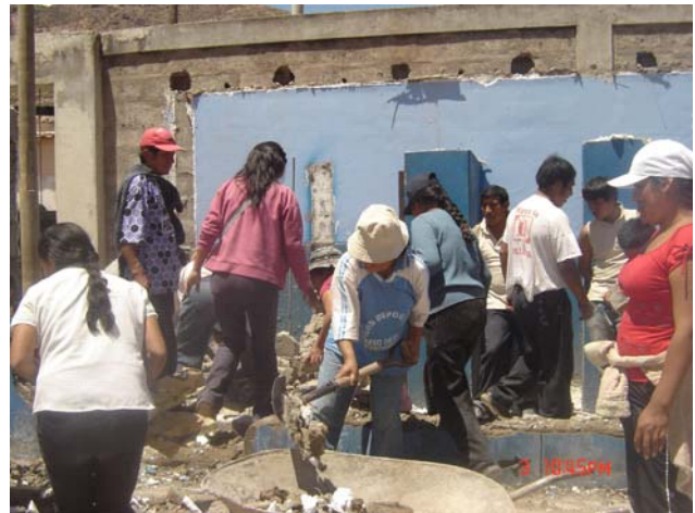
Parents of the school children help with the construction of the new bathroom facilities at their children's school
