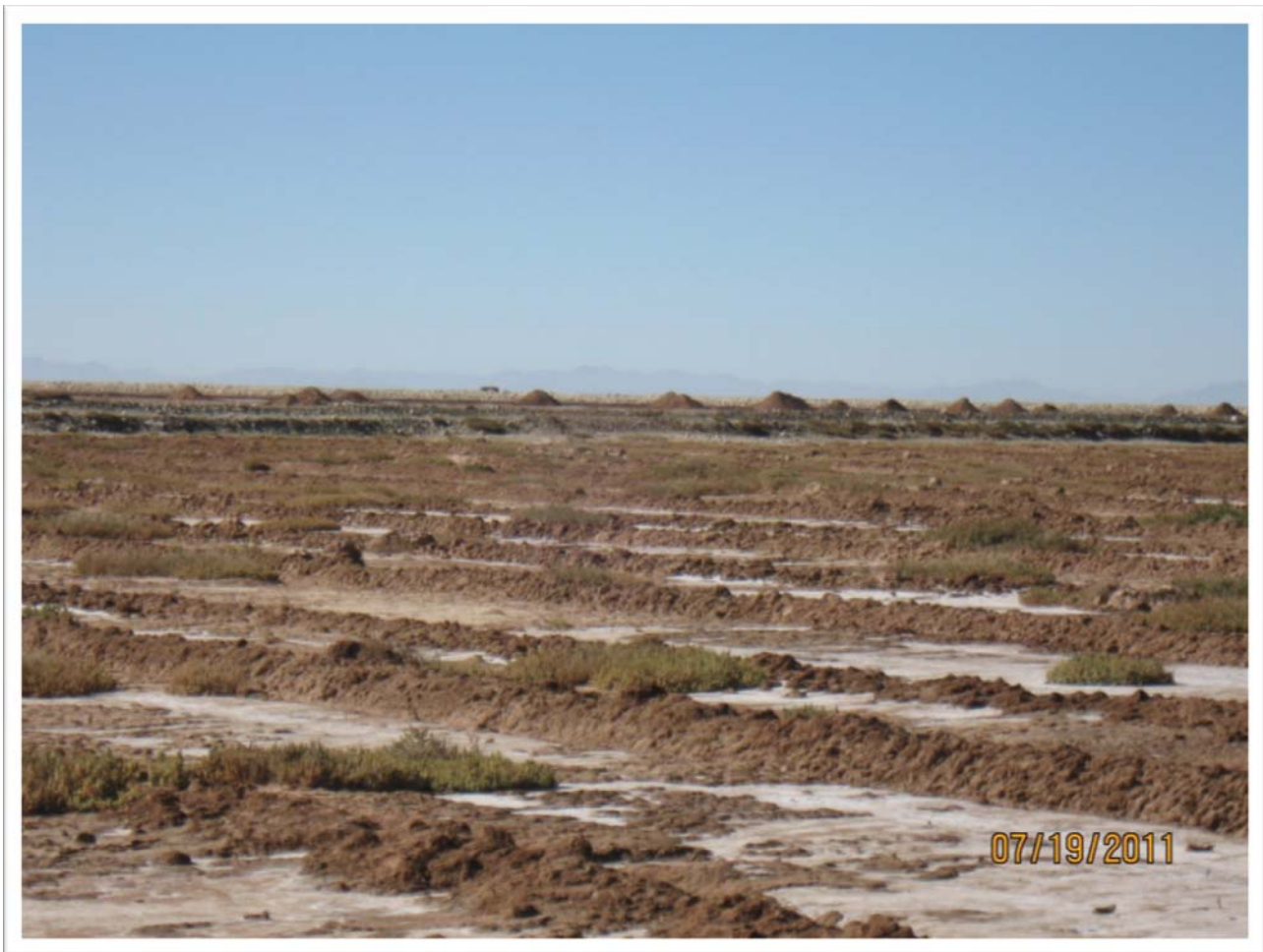
Figure 8 - soil being removed for use as tailings cover, note salt
