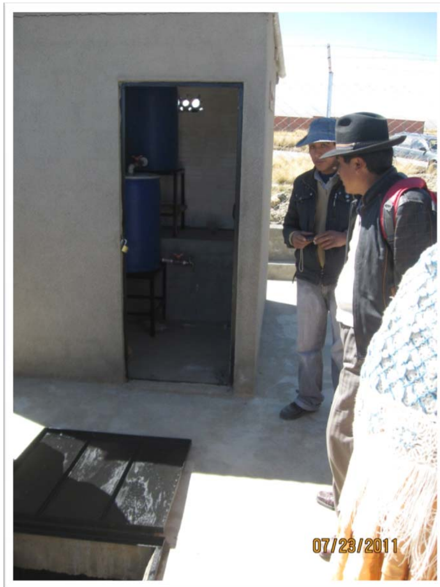
Figure 10 - Machacamarca water storage tank with chlorination system in structure
