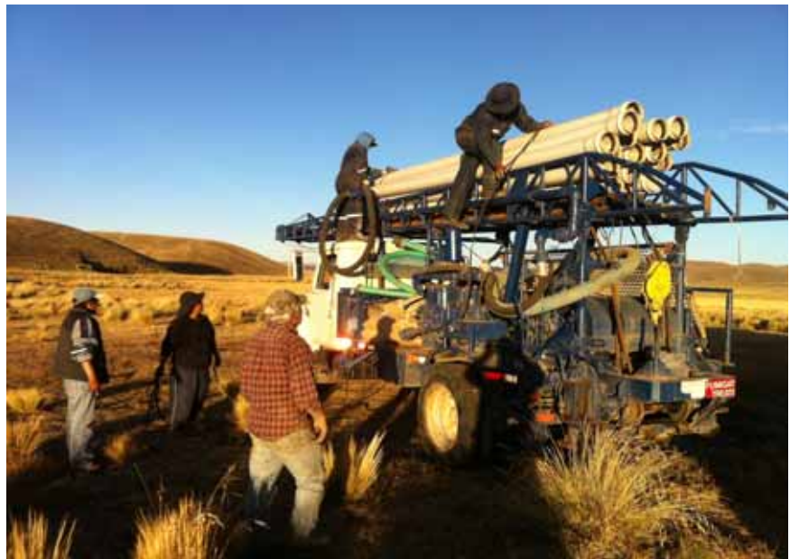
Loading up the rig after the first well
