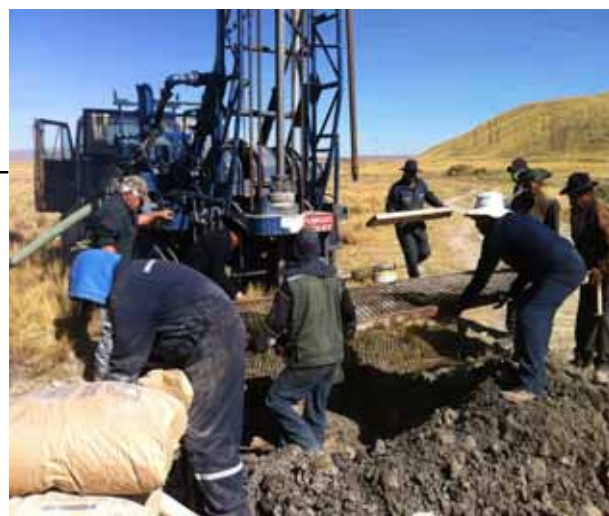
Community members all pitched in to get the drilling started
