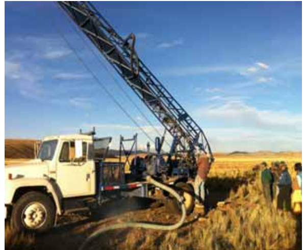
Suma Jayma's water well drilling rig
