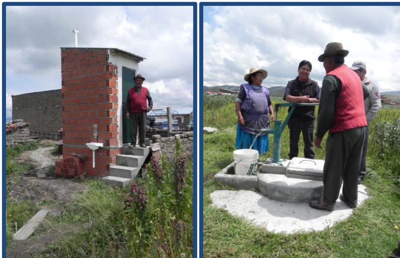
Ecological latrine and manual hand pump and well in Batallas
