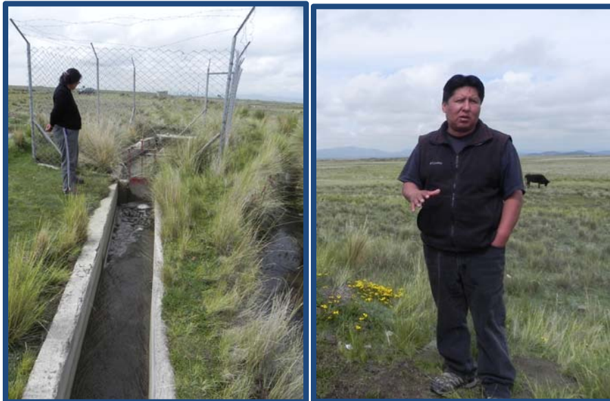
L-Braulio's wife Basilica at the current surface water diversion site structure. R-Braulio explains some history of the Machacamarca project at the underground storage tank
