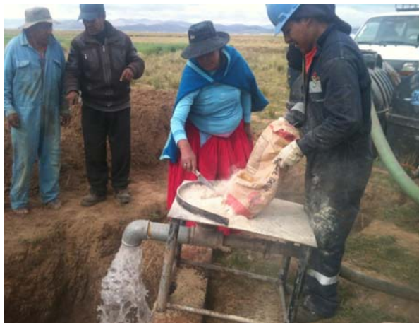
Community members assist the Suma Jayma team throughout the drilling process, including preparation of the drilling mud.
