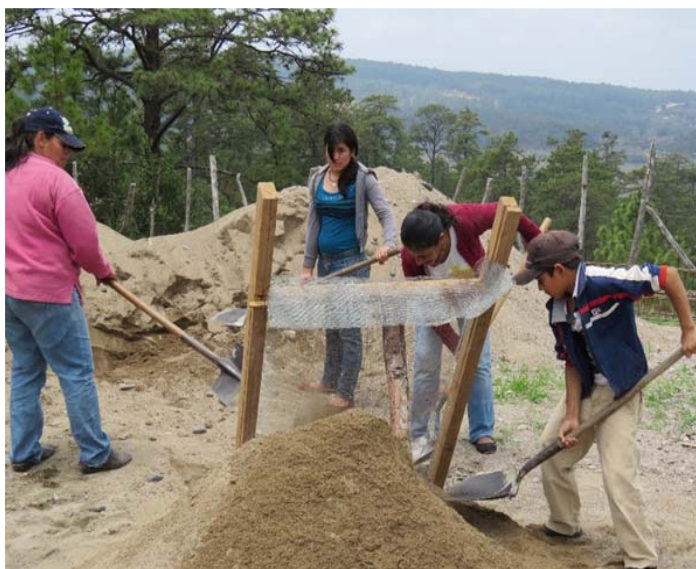
The whole family pitches in preparing sand for the concrete mix.
