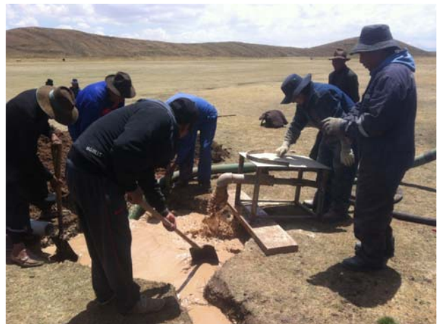
The important task of mixing the drilling mud. One of the ways the locals can help.
