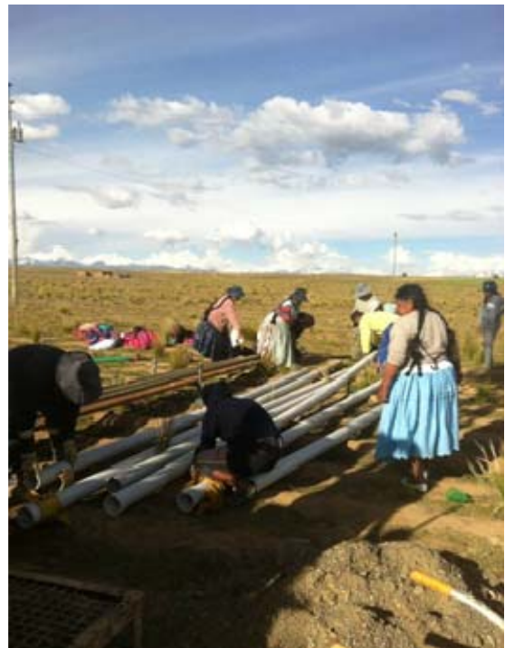
Gathering and preparing the well casing pipe
