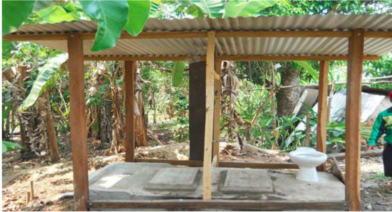
Concrete septic tank with two separate chambers. The toilet is installed over one chamber and the shower is installed over the second chamber
