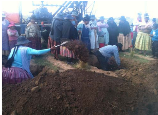
Women and men alike from the community assist with the excavation of the pits to be used to prepare the drilling mud. Hard physical labor is nothing foreign to the Aymaran people.
