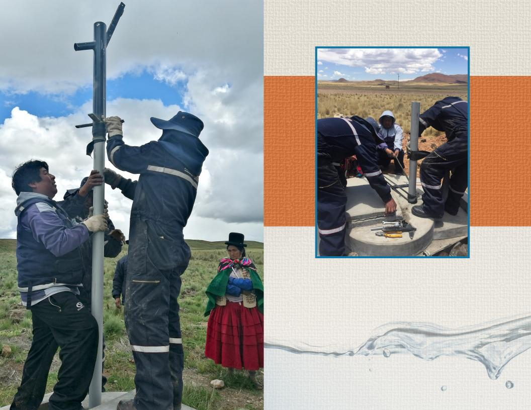
Installation is completed by connecting the fabricated hand pump to the well. Function of the new hand pump is tested by the Suma Jayma team.
