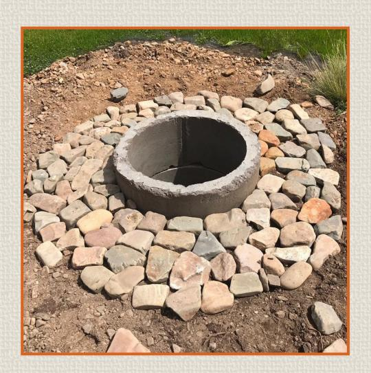
With the concrete rings installed, stones are placed and preparation is made to pour the concrete pad that forms the outer protection of the well.
