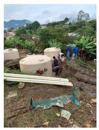
inlets and outlets were cut into each tank using a drill and hole saw bit.
