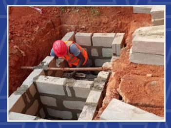
The wastewater system improvements portion of the project included construction of a shallow sewer network with 19 manholes, 36 collection chambers, 16 settling chambers, an Anaerobic Baffled Reactor (ABR), Aerated Composite Filter (ACF), Polishing Tank (PT), and disposal system for the treated effluent below ground into a leach field.
