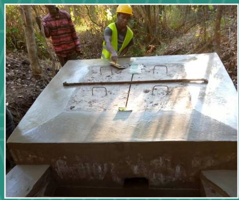
At the river crossing, PVC pipe was replaced with 2" galvanized iron pipe supported by concrete columns to protect the transmission line from flooding.
