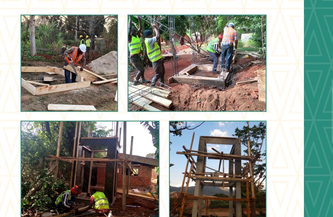
Two new concrete tank towers were constructed to provide additional water storage and adequate water pressure for St. John's Hospital and the Sisters' Convent.
