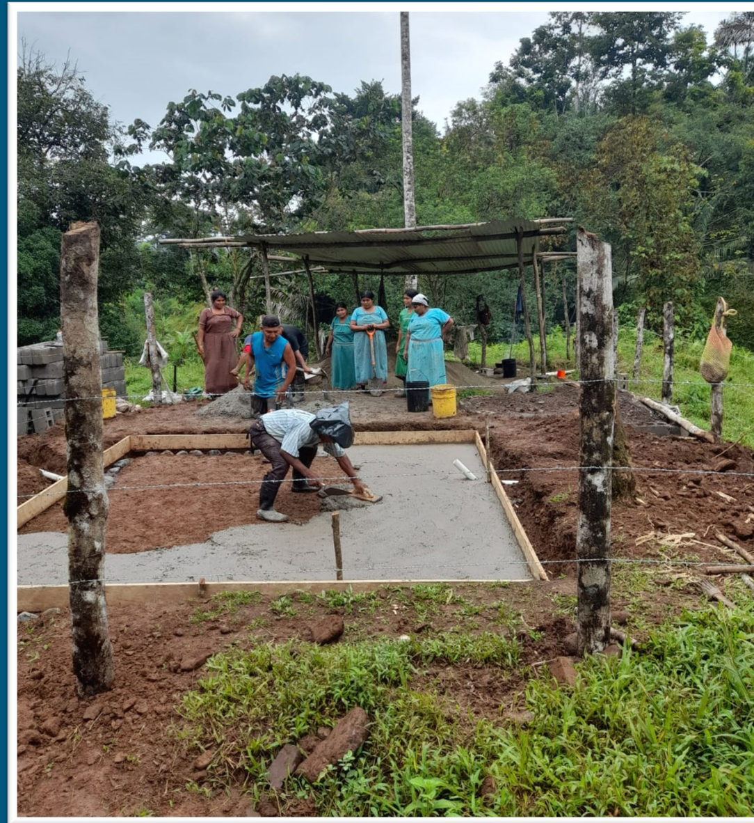
The water storage tank site is cleared and leveled. The bottom slab is poured and finished.
