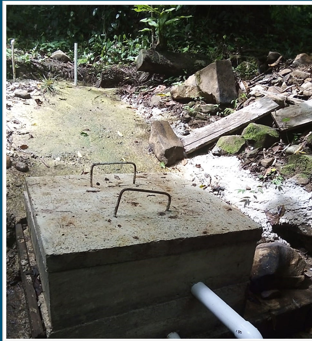
The old spring capture was leaking from underneath the capture foundation, and beyond repair. José worked with the junta to completely rebuild the spring capture
