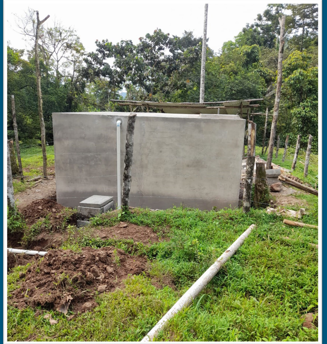
The tank is complete. Outlet valves are protected with valve boxes and the outlet is connected to the distribution system.
