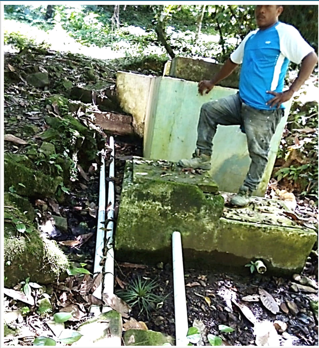
The old spring capture was leaking from underneath the capture foundation, and beyond repair. José worked with the junta to completely rebuild the spring capture
