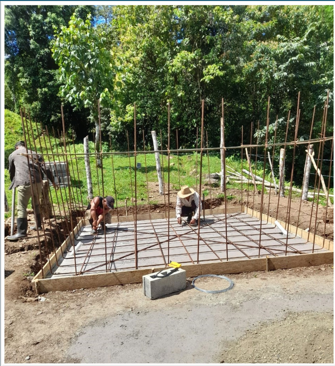
Steel re-bar is laid out for the final slab pour and the beginning of the tank walls.
