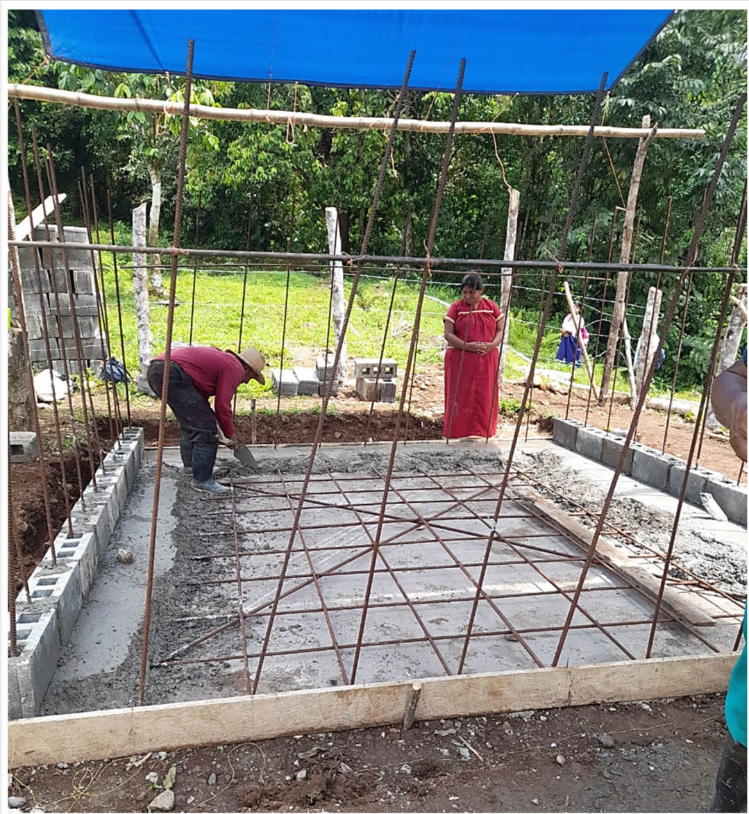
The final tank floor is poured and finished. Steel Re-bar wraps around the tank on block courses to reinforce the tank walls.
