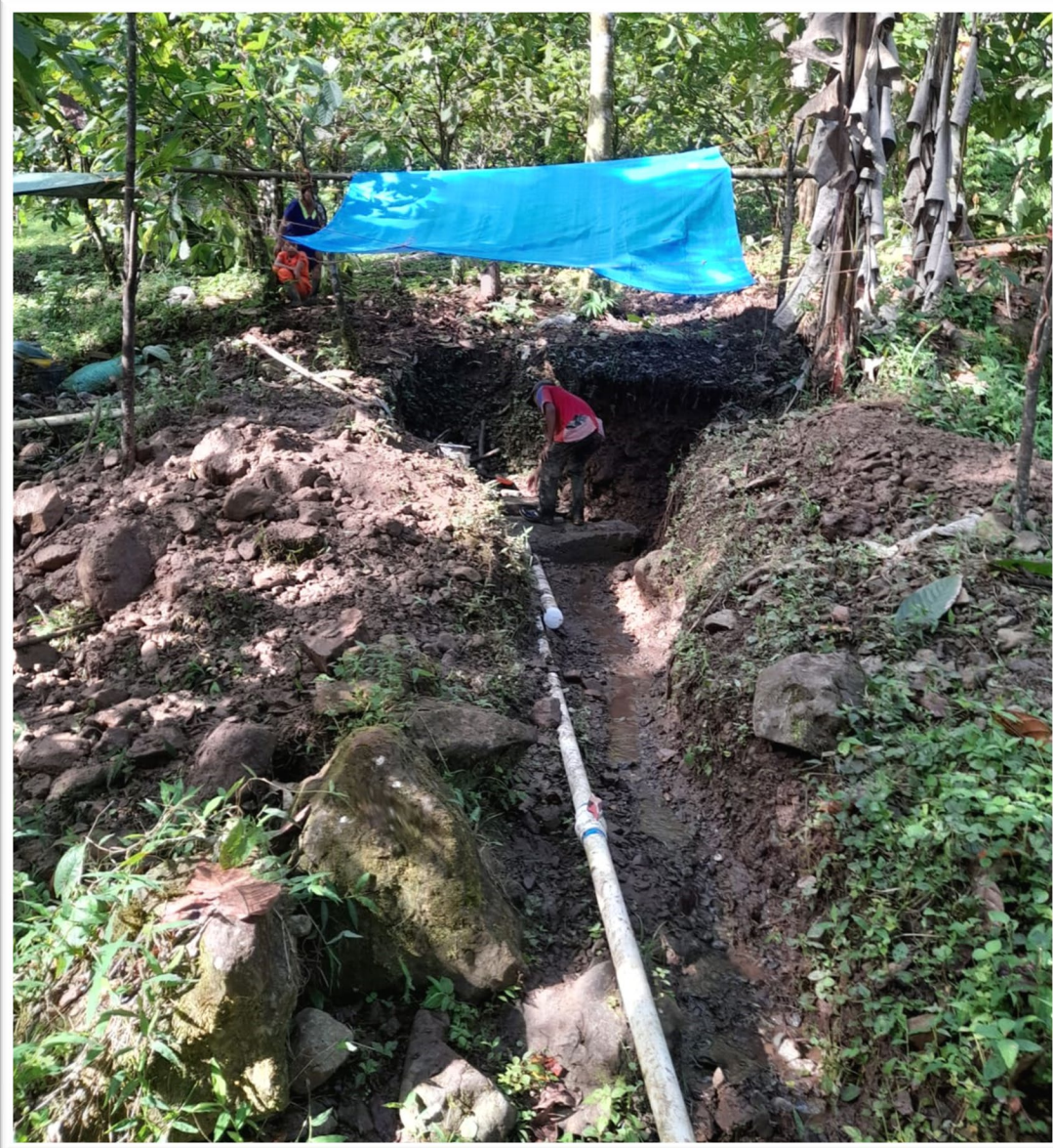
The spring source is captured and protected, then piped to the community via the transmission line.
