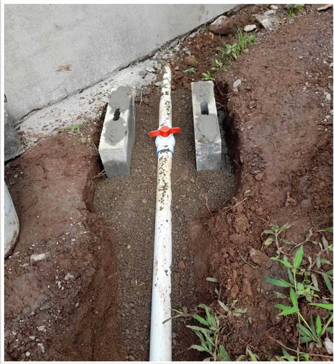
The tank is complete. Outlet valves are protected with valve boxes and the outlet is connected to the distribution system.
