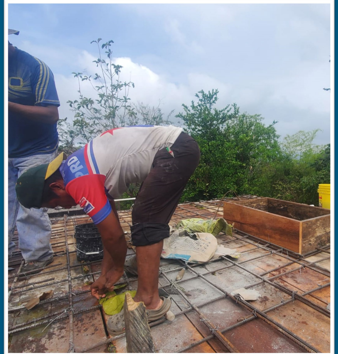
The tank ceiling/roof is supported and reinforced with rebar for the concrete pour. A tank hatch is built to allow for access in and out of the tank for cleaning.
