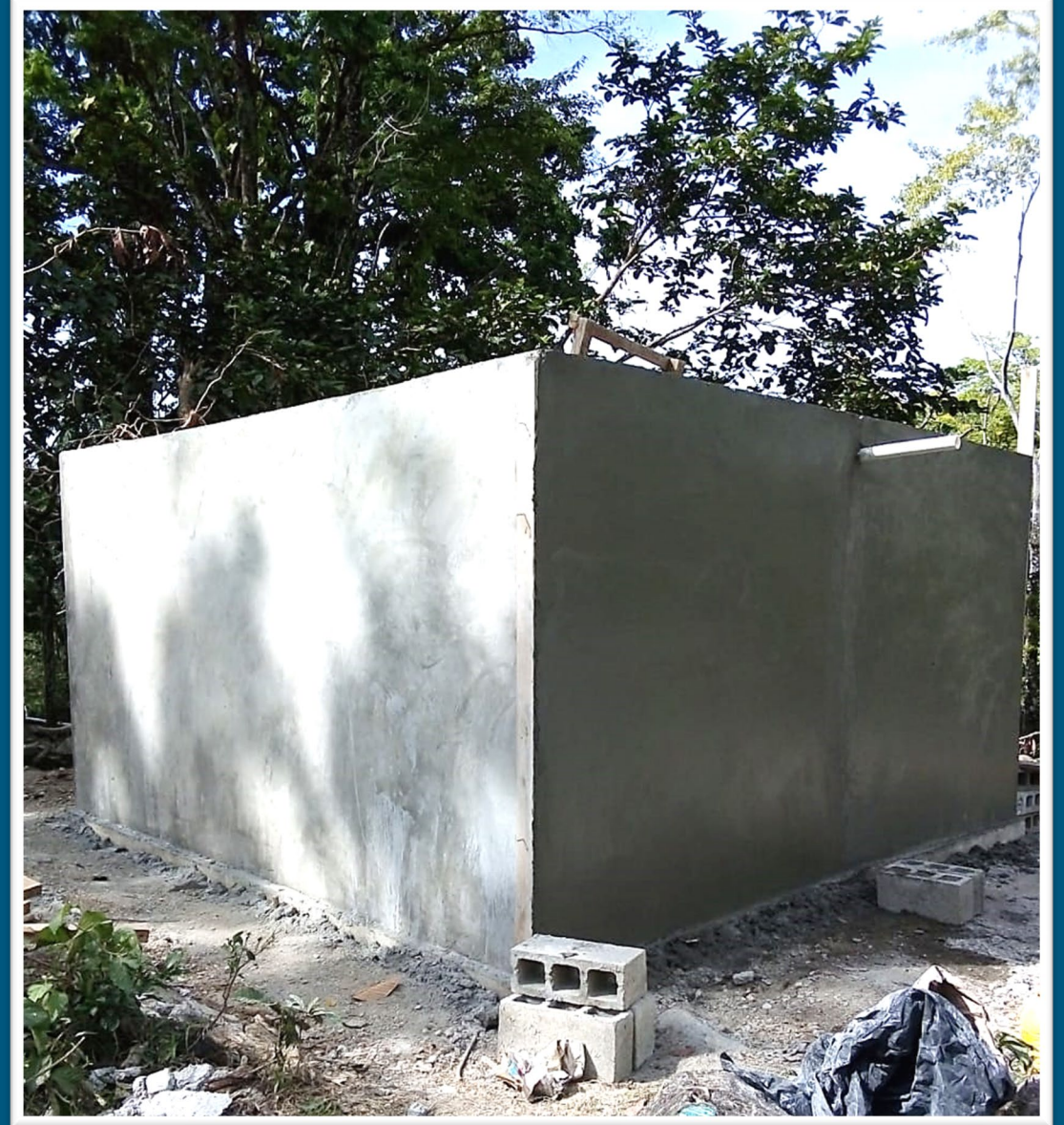
The original water system had three plastic tanks for water storage. They all leaked and were insufficient for storage. A new tank was built on site. The old tanks were repair and placed at the school for rainwater collection.
