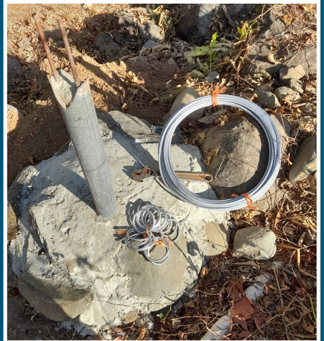
The community and Nicolas work to repair the existing waterline bridge crossing. Steel cable and reinforced anchors are used to keep the waterline above the flood level of the stream.
