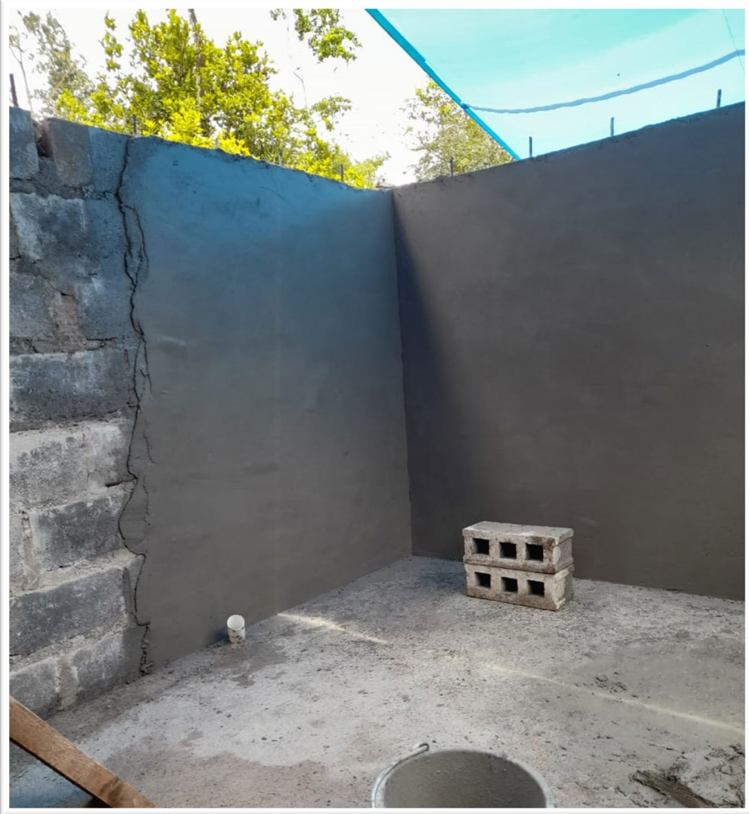
Once the tank walls are complete, the walls are plastered to be waterproof inside and out.
