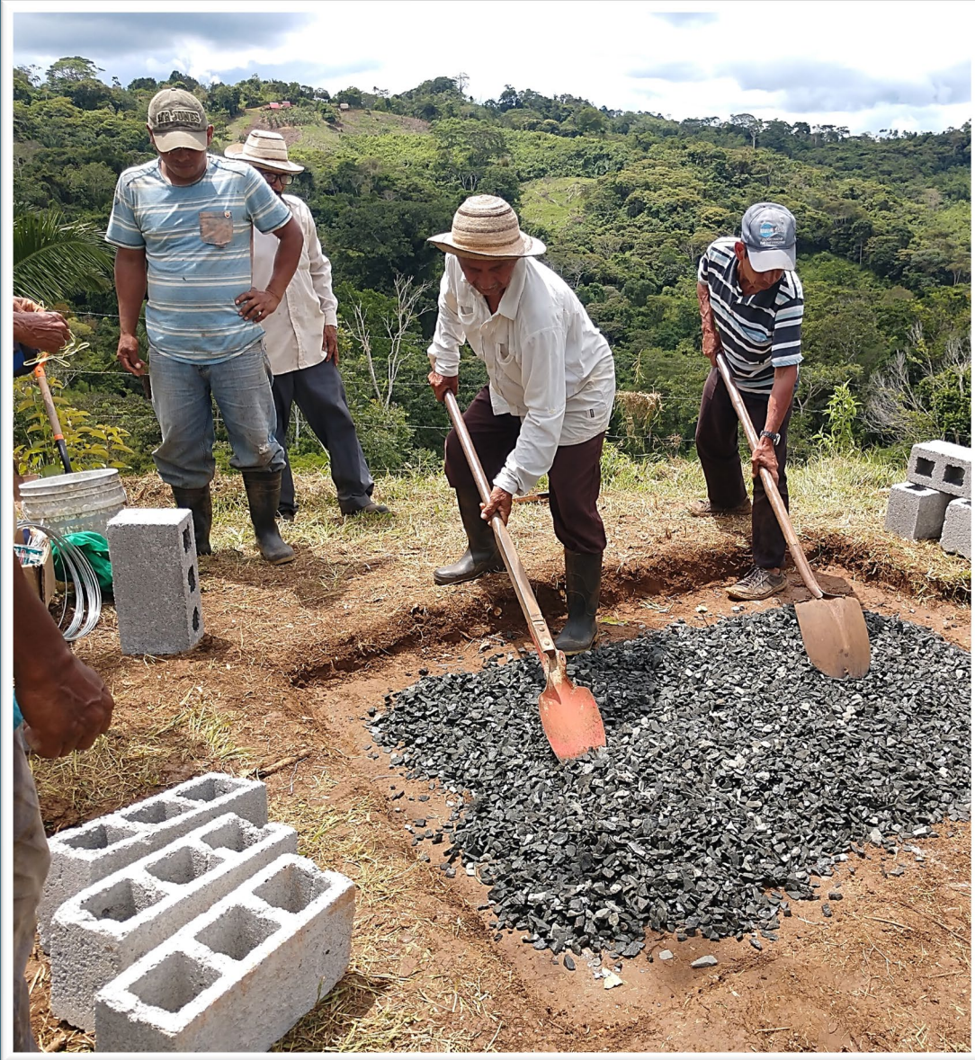
The break pressure tank site is prepared for the first concrete pour of the floor.
