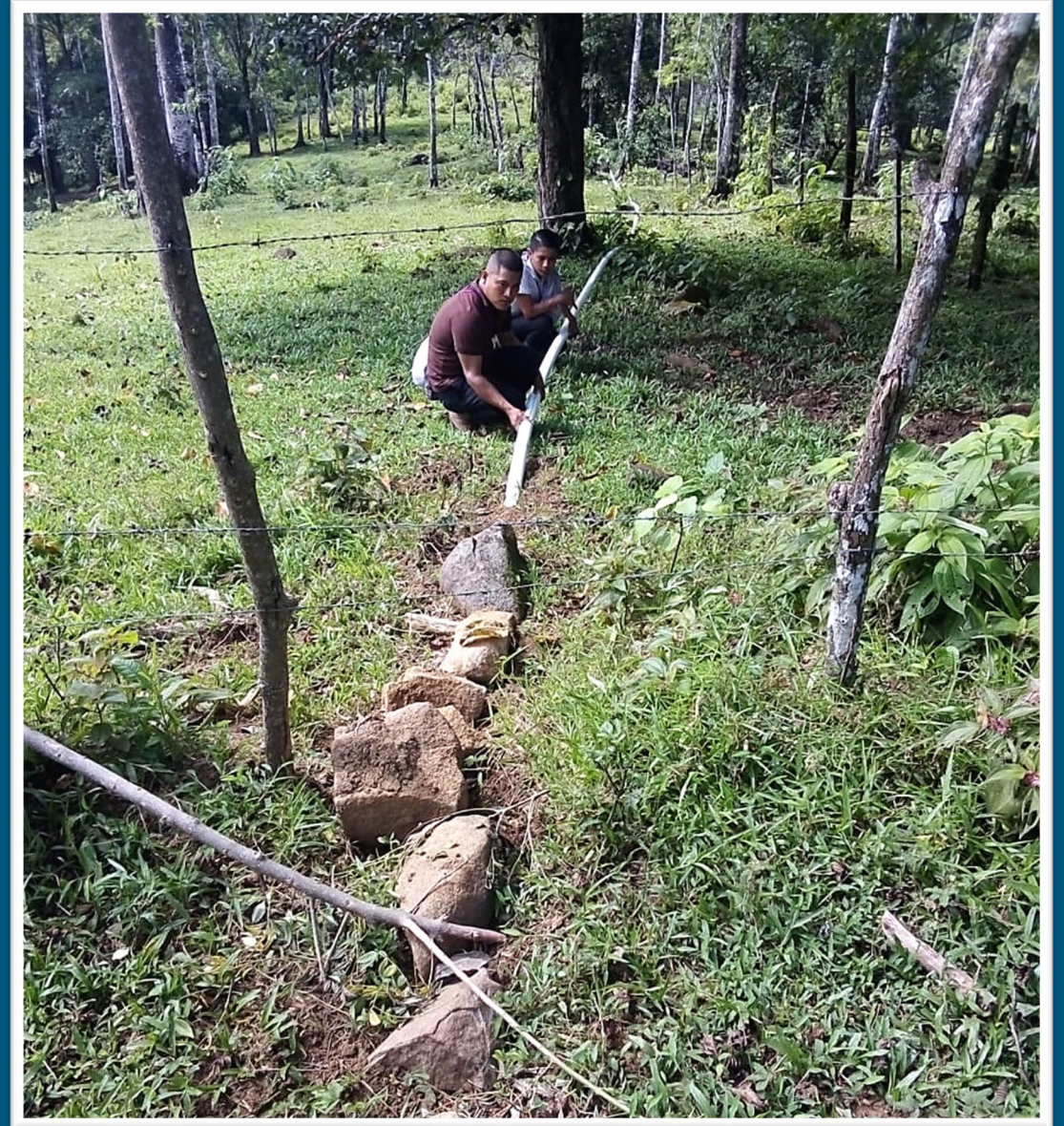
A new transmission line was installed. Rocks cover the line where the soil is too rocky to bury the line. Shut off valves and valve boxes are installed to control water flow.
