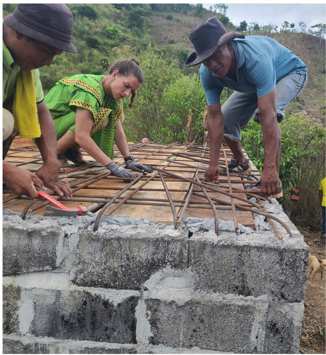
The tank ceiling/roof is supported and reinforced with rebar for the concrete pour. A tank hatch is built to allow for access in and out of the tank for cleaning.
