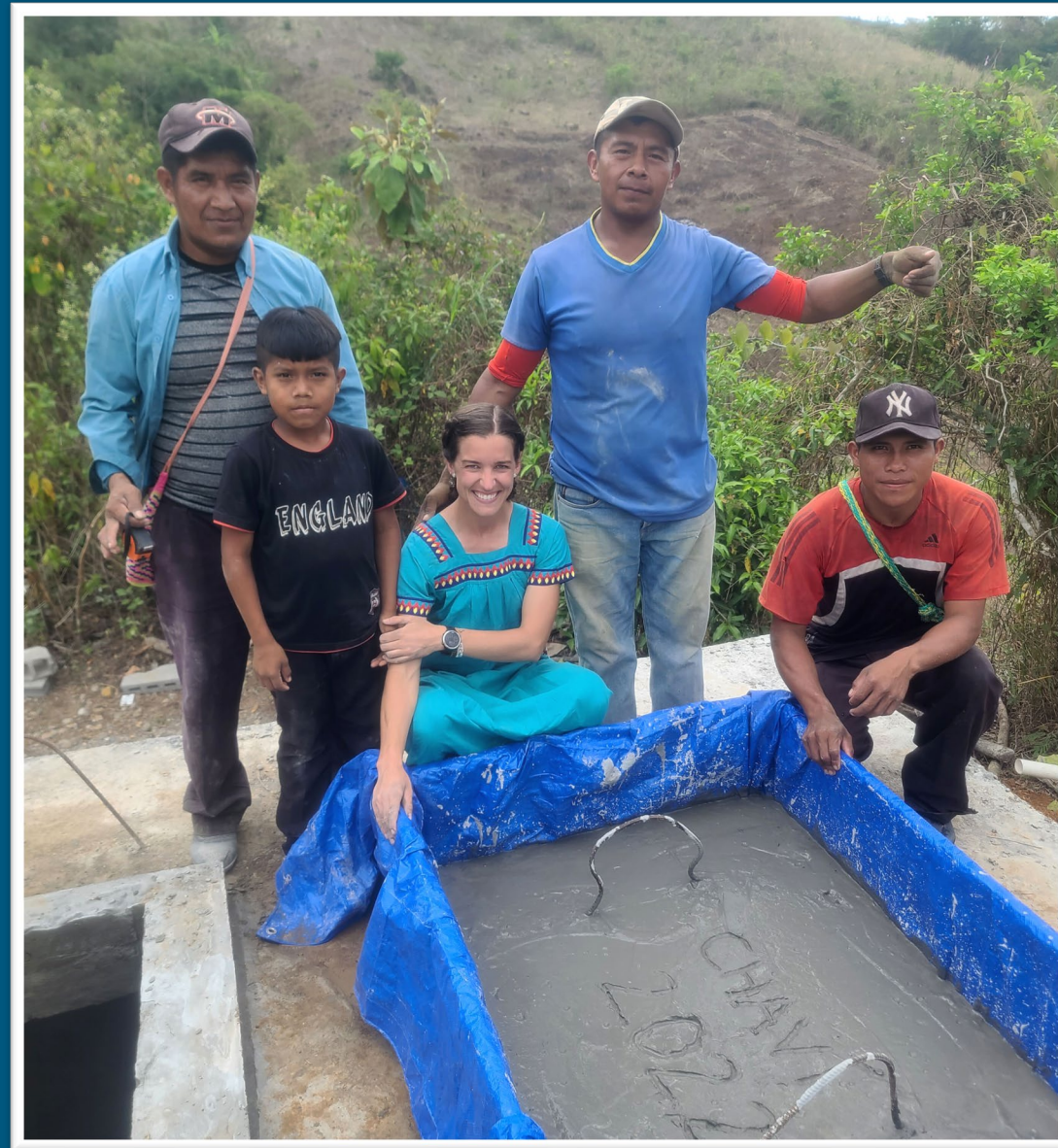
The community and WEFTA volunteers work together. The water storage tank is complete with a lid for the access port.
