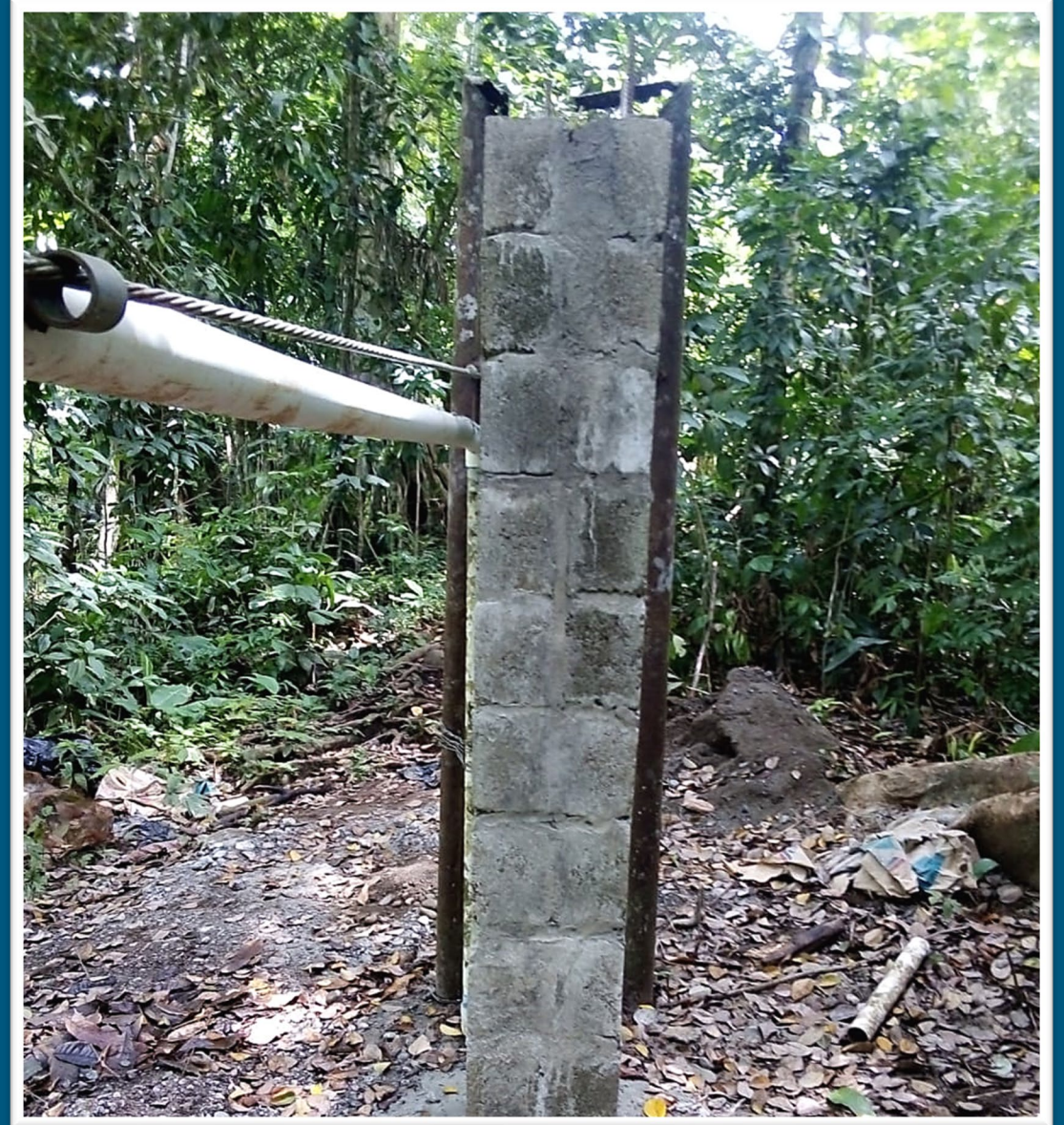
Where the original bridge structure was rusted and failing, a new block pillar was constructed to support the transmission line over large creek crossings.
