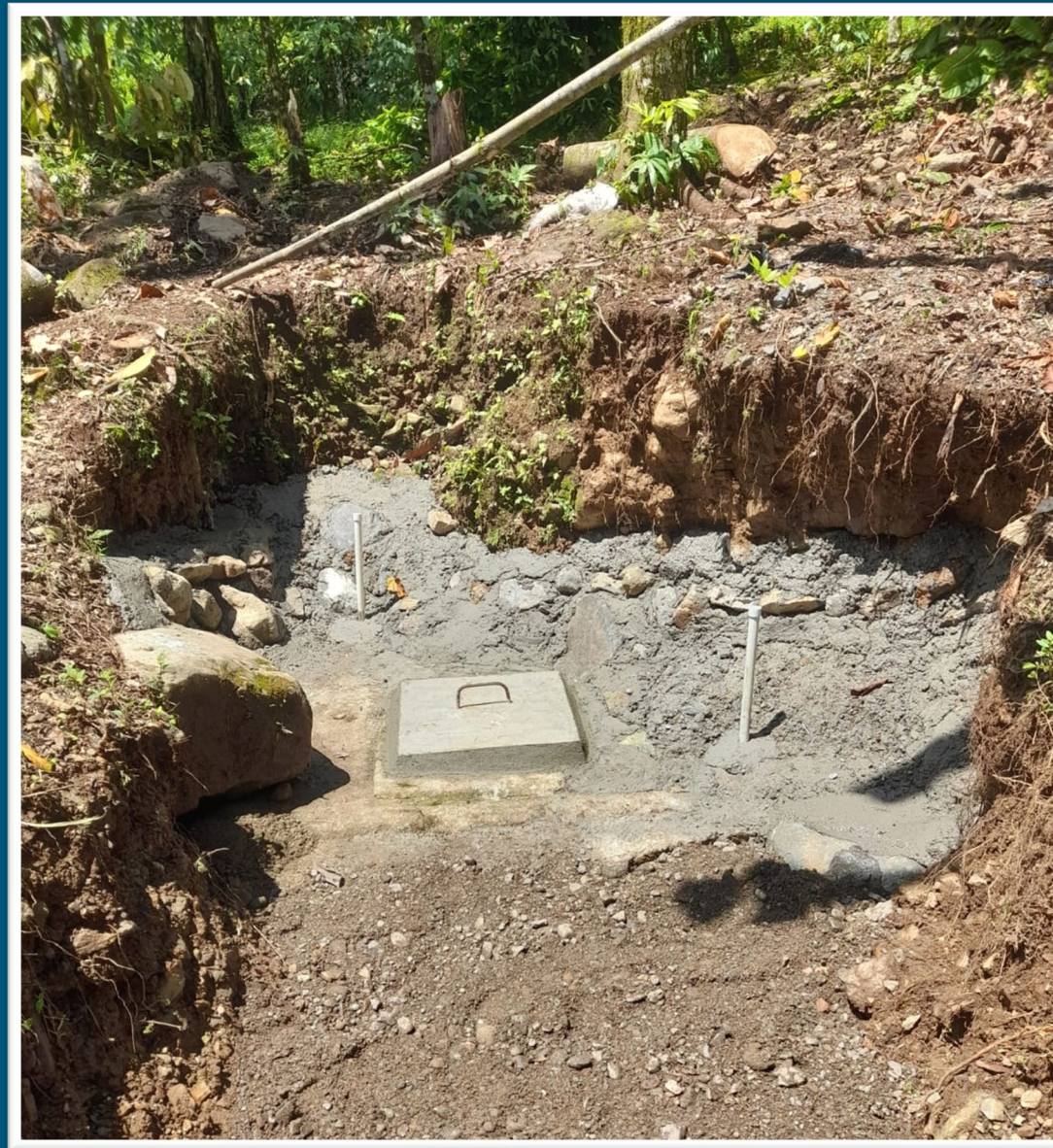
The spring source is flowing well. The spring capture area is complete.
