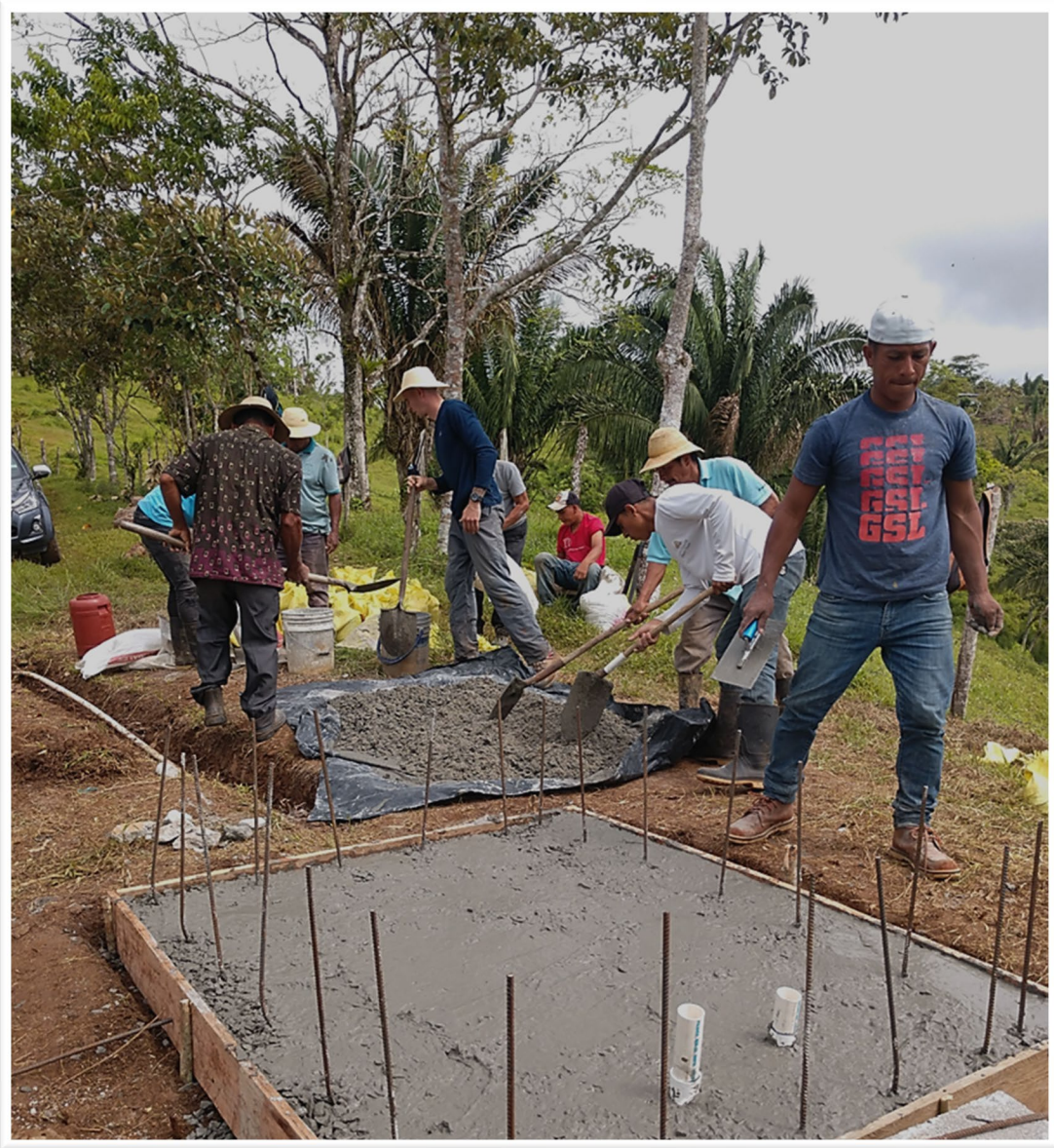
The floor is finished. Blocks and steel re-bar make up the tank walls.
