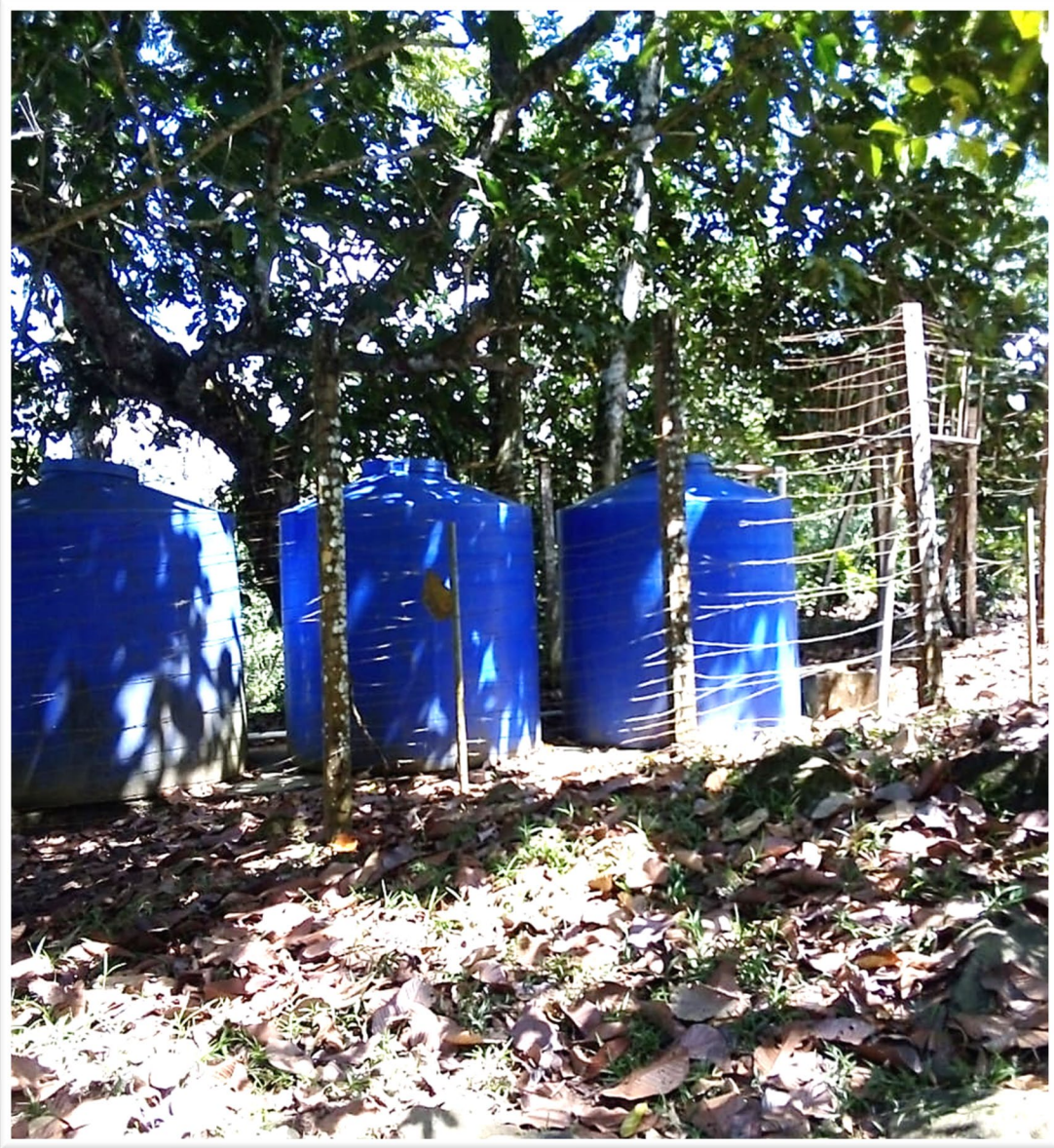
The original water system had three plastic tanks for water storage. They all leaked and were insufficient for storage. A new tank was built on site. The old tanks were repair and placed at the school for rainwater collection.
