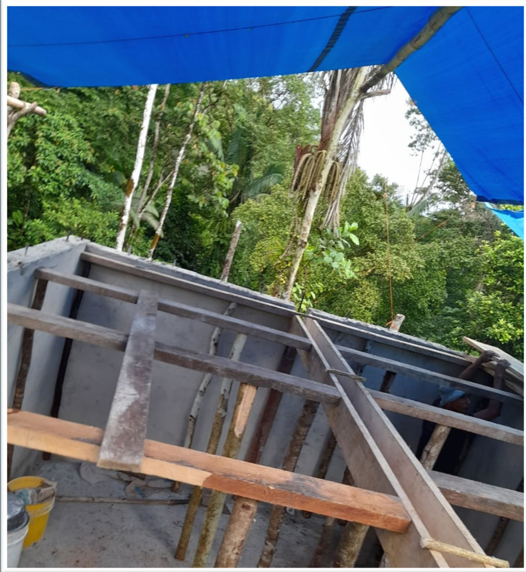
The tank ceiling is formed, supported, and rebar is tied in to complete the total tank reinforcement. The tank ceiling is then poured.
