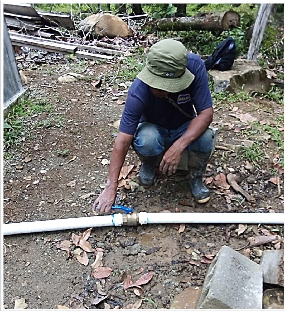
A new transmission line was installed. Rocks cover the line where the soil is too rocky to bury the line. Shut off valves and valve boxes are installed to control water flow.
