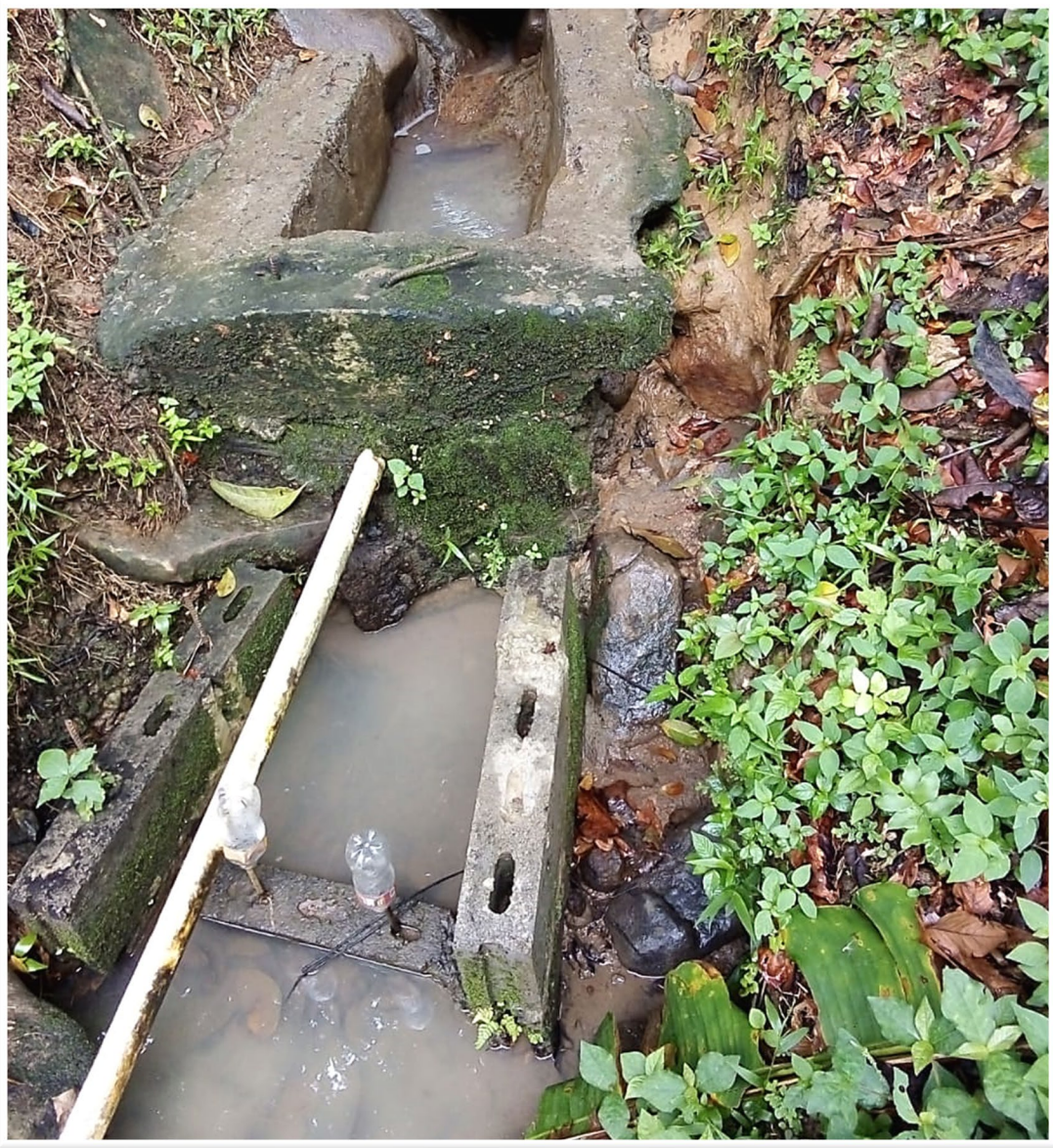
The second spring capture was also in complete disrepair. The junta and José built a brand-new spring capture – in Panama it is called a 'toma'.
