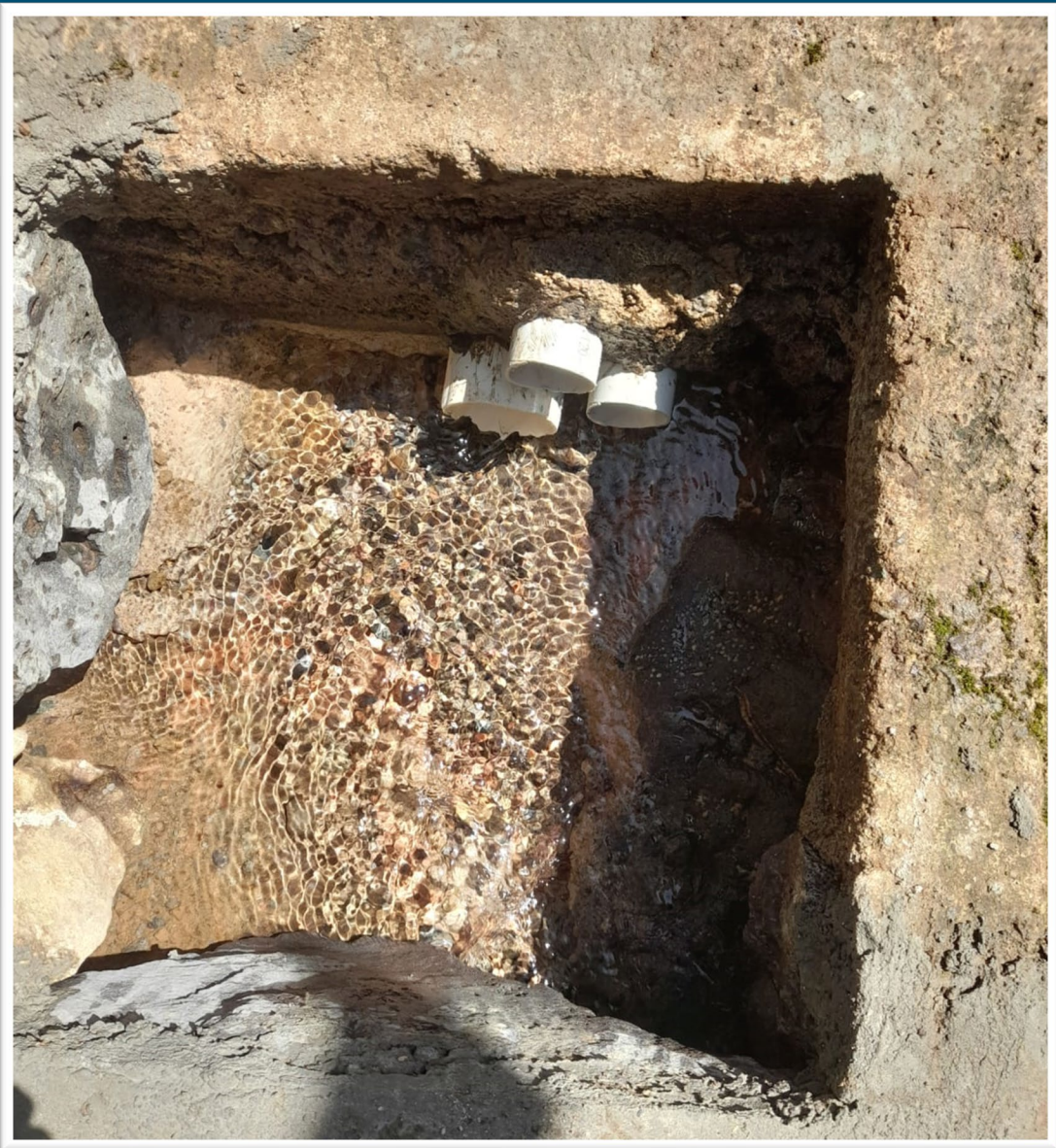
The spring source is flowing well. The spring capture area is complete.
