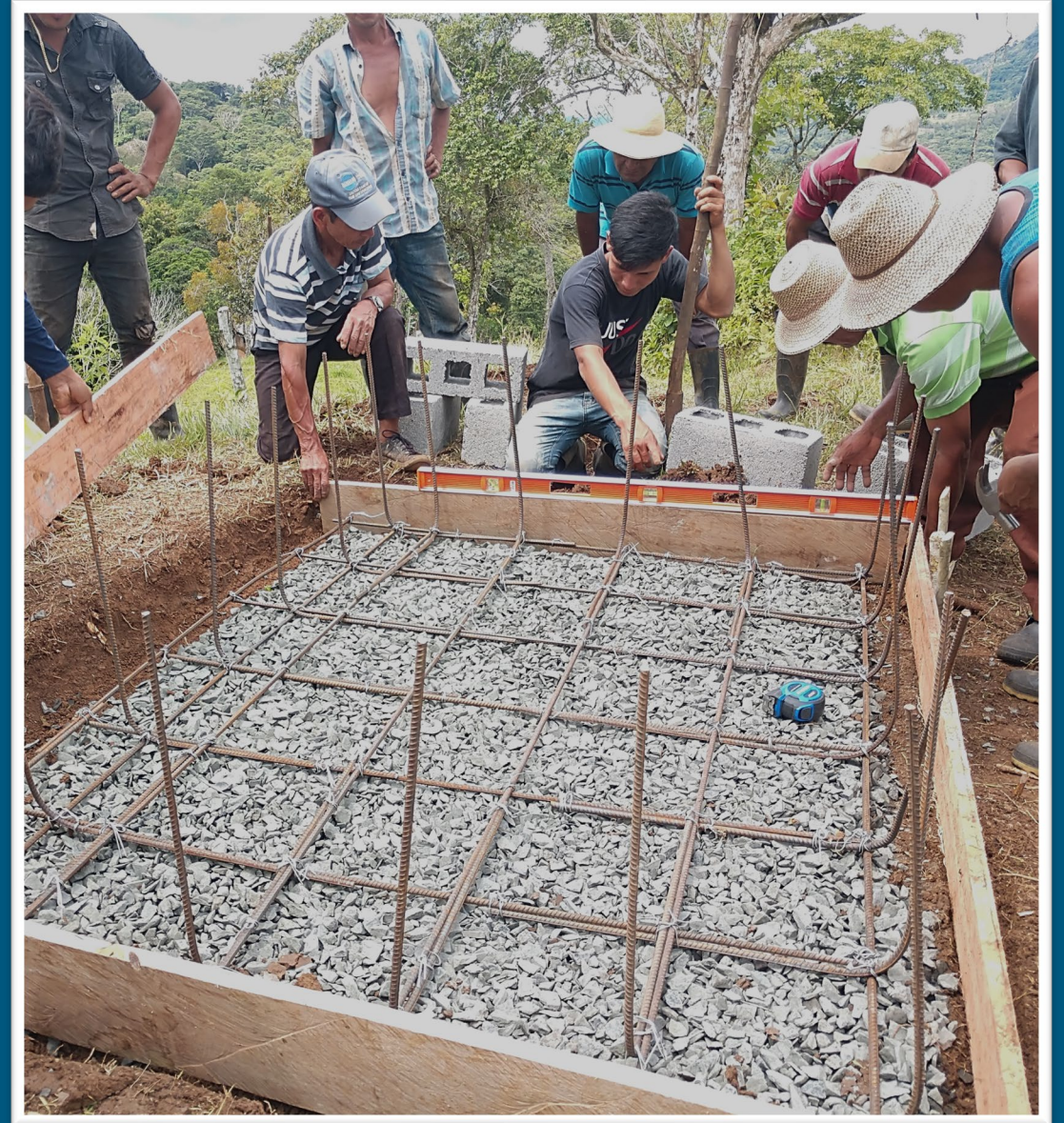
The break pressure tank site is prepared for the first concrete pour of the floor.
