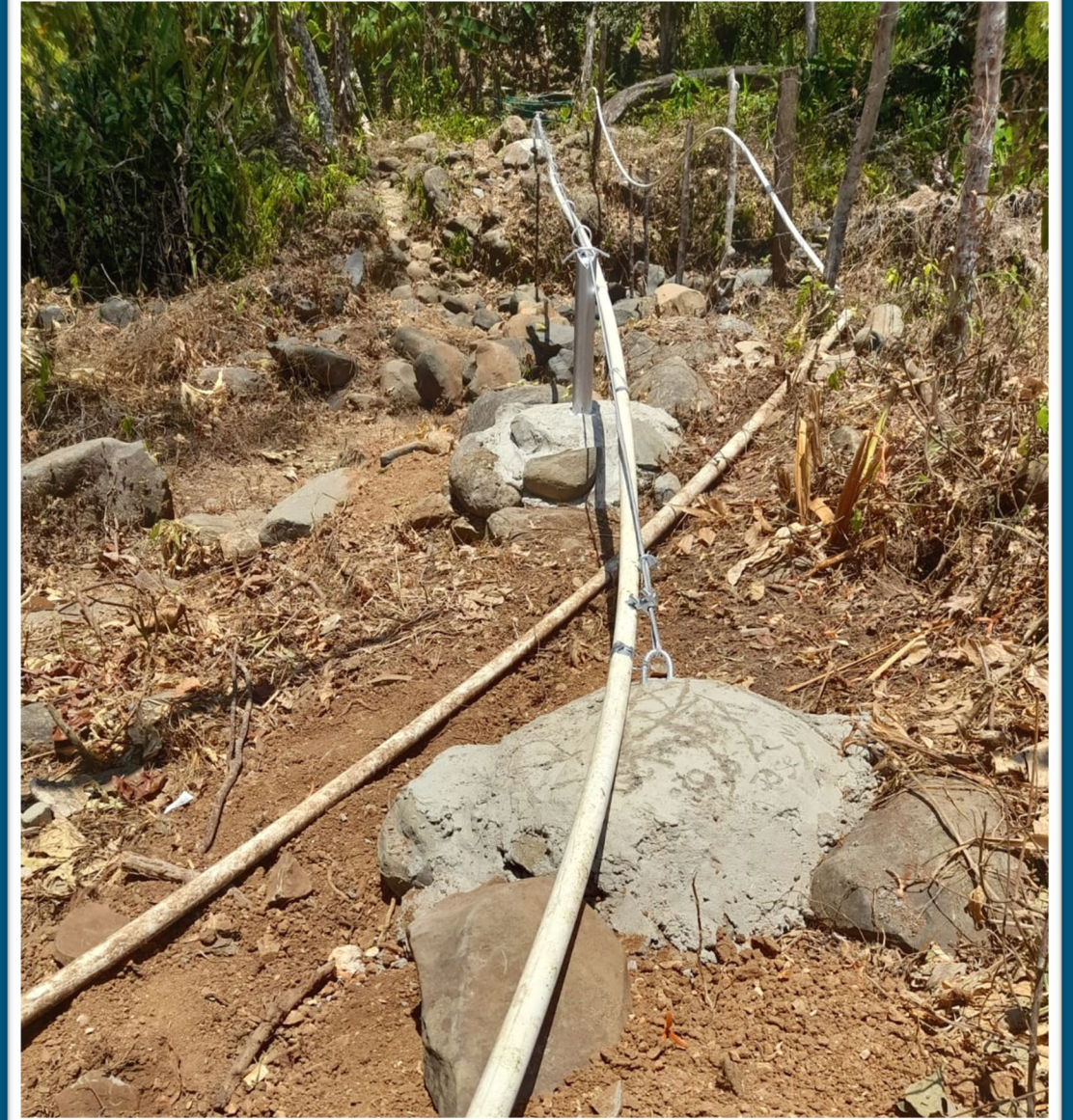
The anchors are set, and the cable is drawn tight. The new waterline is connected to the cables and will be painted to prevent sun damage.
