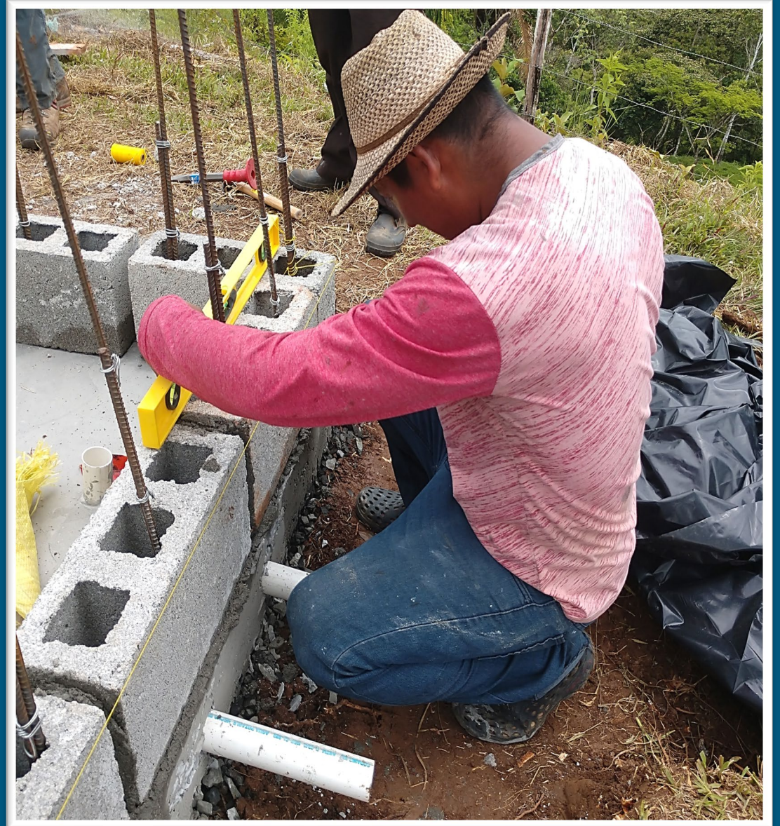
The floor is finished. Blocks and steel re-bar make up the tank walls.
