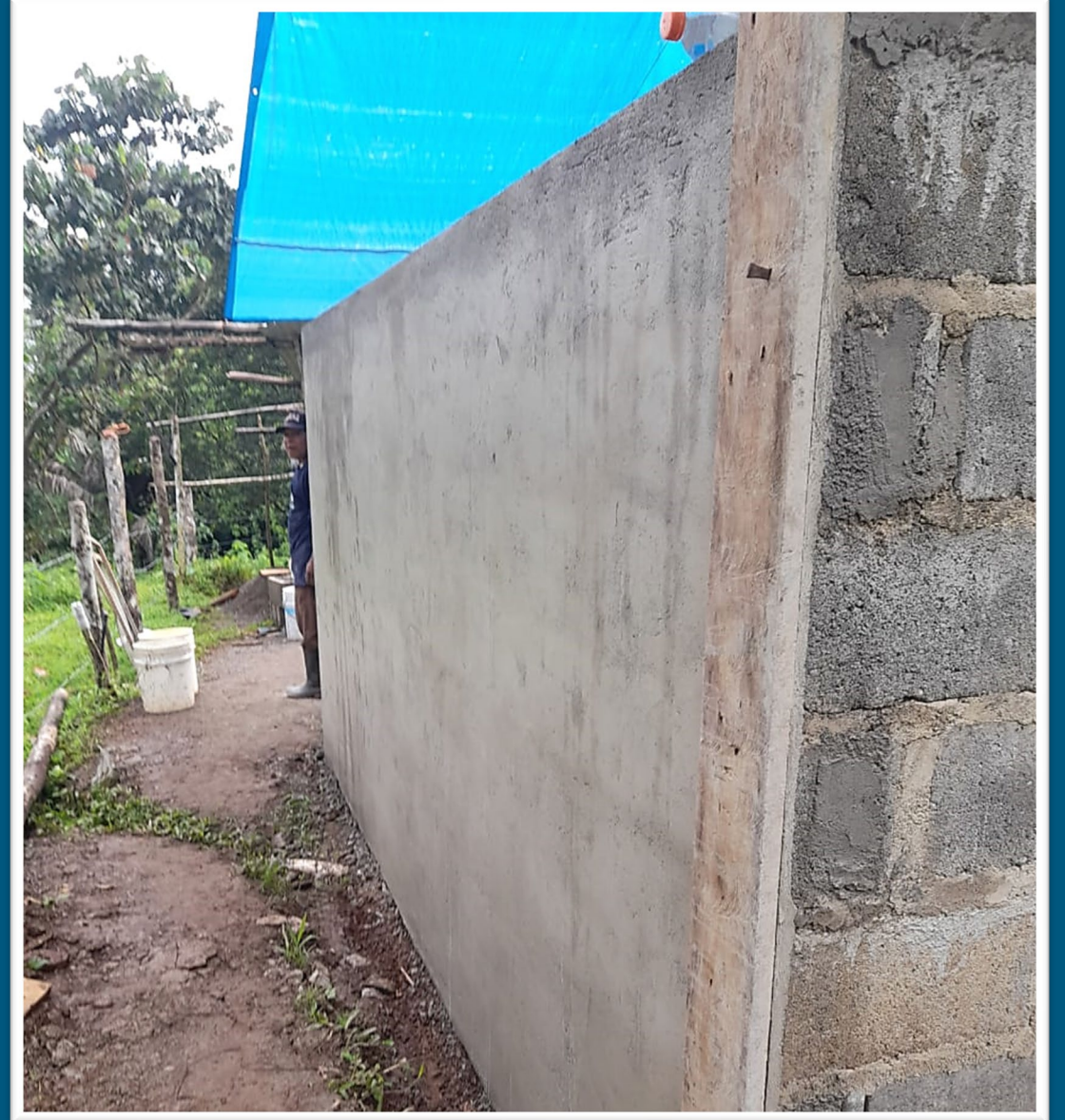
Once the tank walls are complete, the walls are plastered to be waterproof inside and out.
