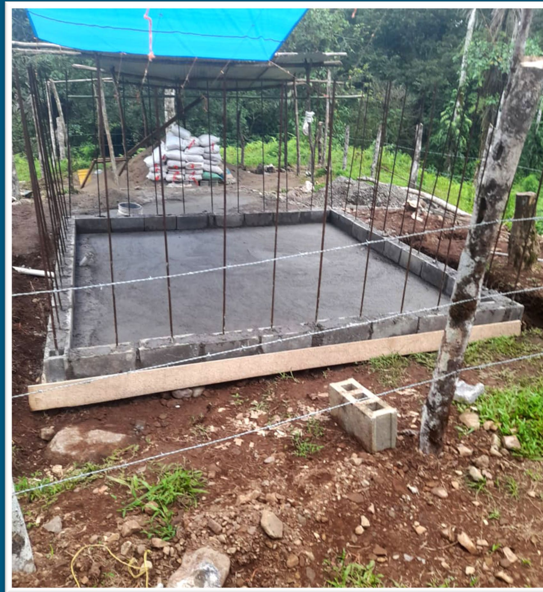
Steel re-bar is laid out for the final slab pour and the beginning of the tank walls.
