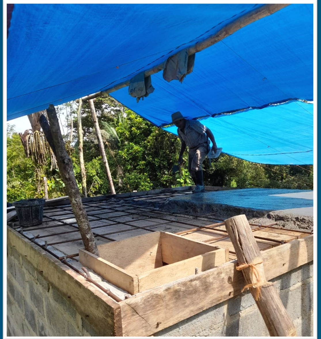
The tank ceiling is formed, supported, and rebar is tied in to complete the total tank reinforcement. The tank ceiling is then poured.
