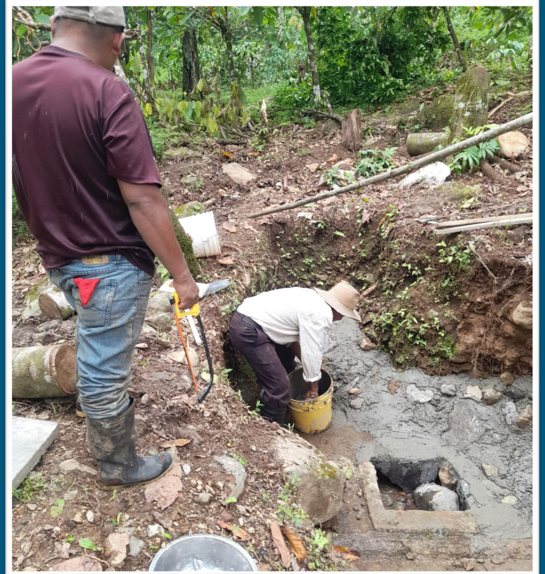
The spring source is captured and protected, then piped to the community via the transmission line.
