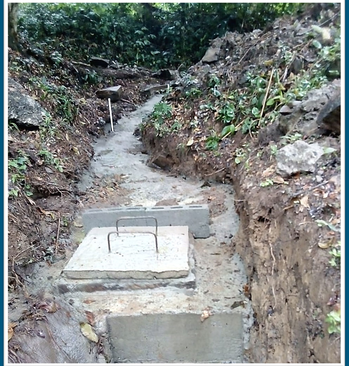
The second spring capture was also in complete disrepair. The junta and José built a brand-new spring capture – in Panama it is called a 'toma'.
