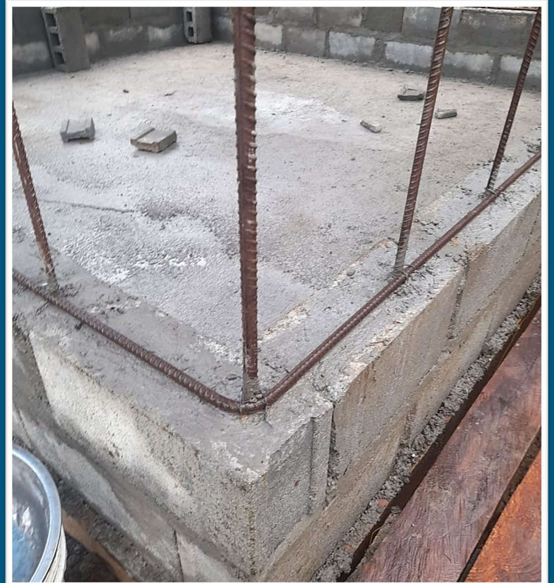
The final tank floor is poured and finished. Steel Re-bar wraps around the tank on block courses to reinforce the tank walls.
