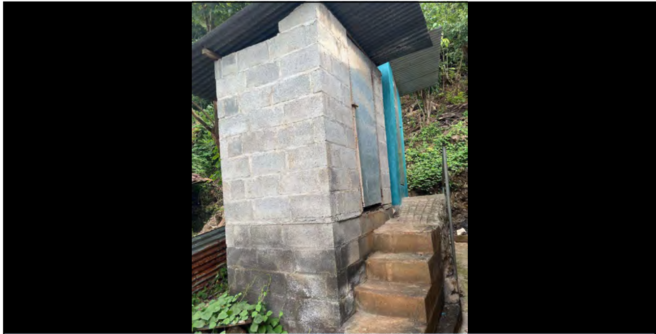
Dry composting latrines are used in areas of high groundwater or where pit latrines do not work. The community of Olomeguita all use composting latrines. There is need to renovate some of the latrines due to overall age.
