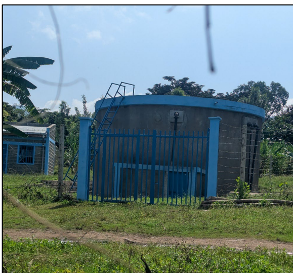
Figure 7: New 50,000 L Storage Reservoir next to Tum Health Center Constructed by the Government
