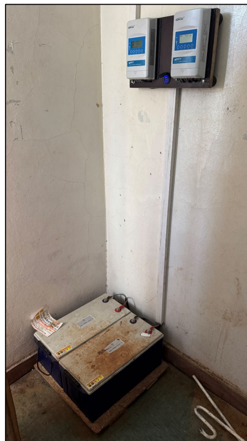
Figure 13: 460W System at Jomu with dirty batteries due to people stepping on them to reach the phone charging port. (Typical of all small systems at the health centers.)
