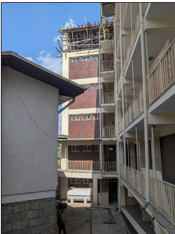
Figure 20: Construction of Water Tower atop New Building
