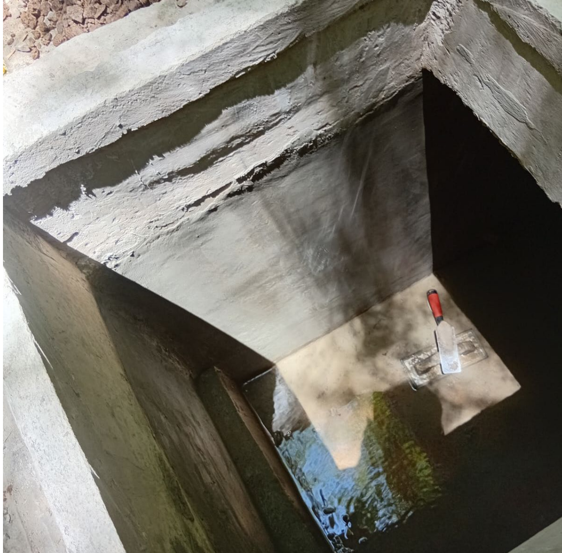
Spring box renovation at the Marogil Spring.
