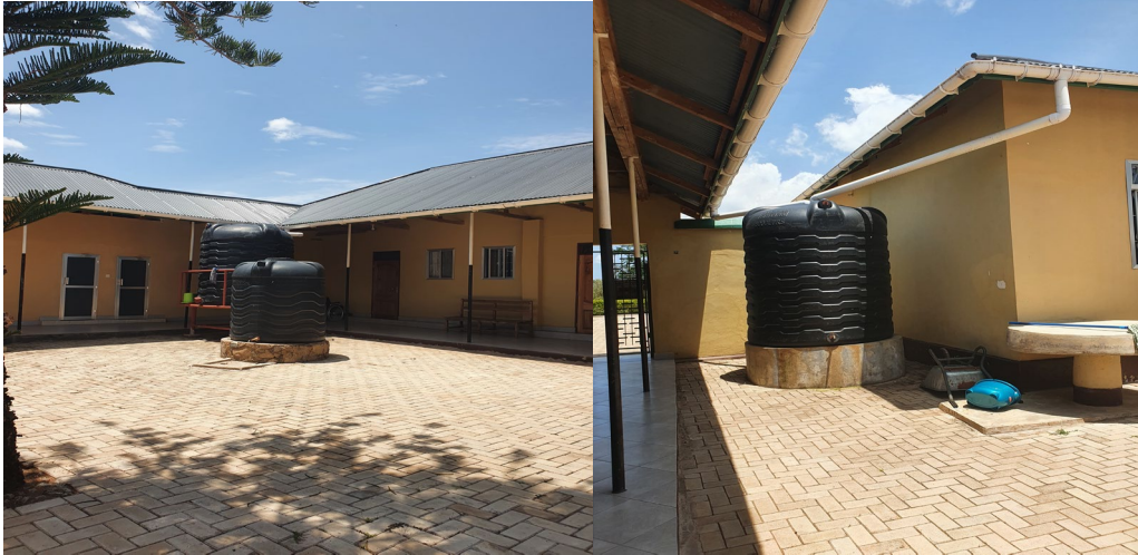
RWH tanks at the HCF Baraki
