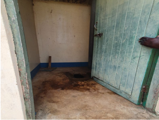
Pit latrine outside the Health care facility
