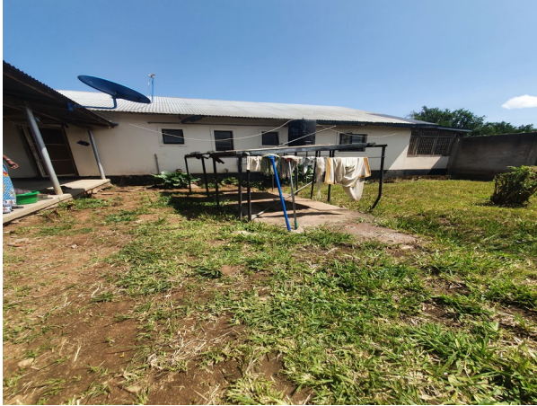
Photo showing solar system for hot water at sisters house Baraki farm built on top of the septic tank
