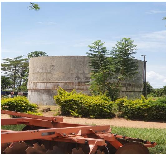
Water Tank that receives water from the lake. It is raised on the base of about 2m
