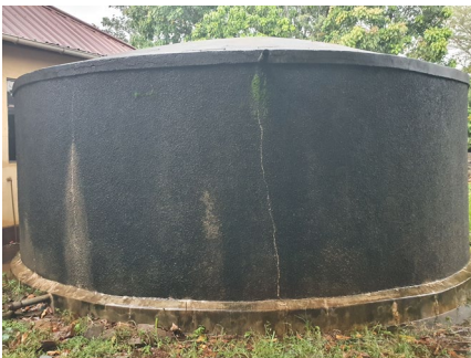
Ferrocement tank for RWH at sisters' convent who are working at Kitenga dispensary
