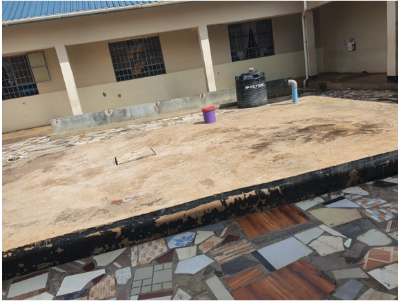
Underground RWH tank at the St Rita of Casia dormitory
