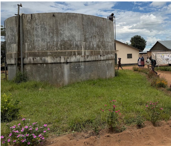
Existing storage tank on a short riser
