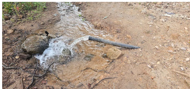
Overflow from Lundu Storage tank
