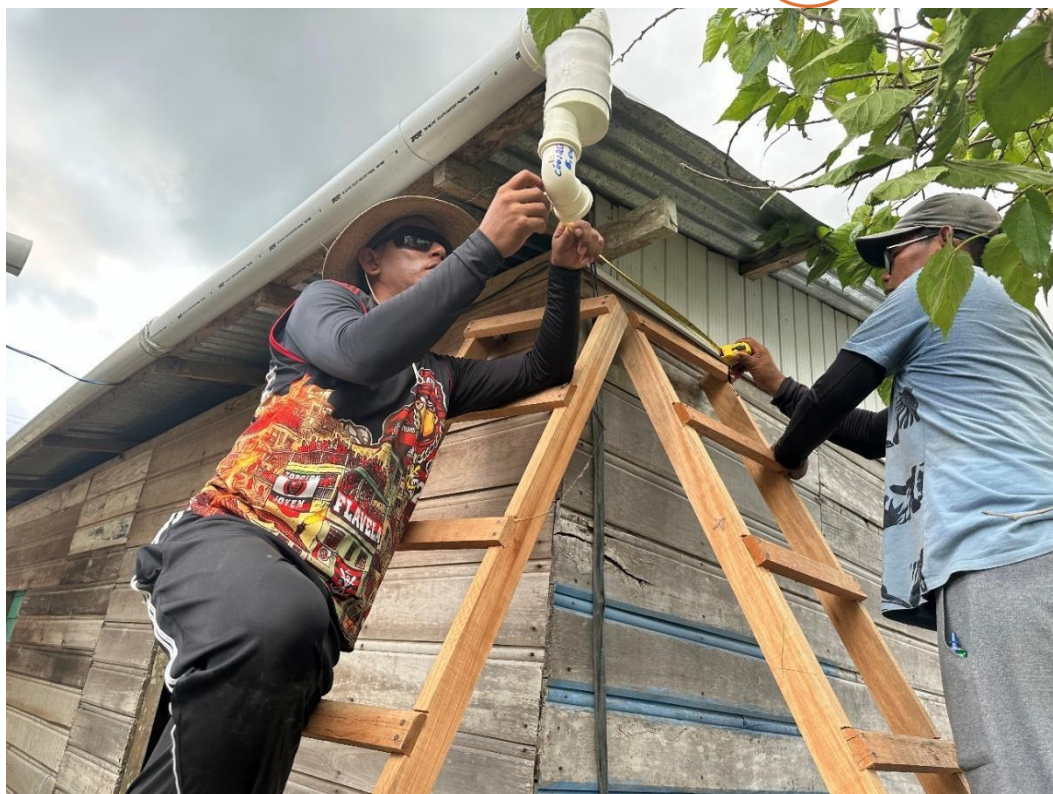
Image 1.11. Technical personnel installing the fittings and routing pipe to the filtration system, Villa Olivença.
