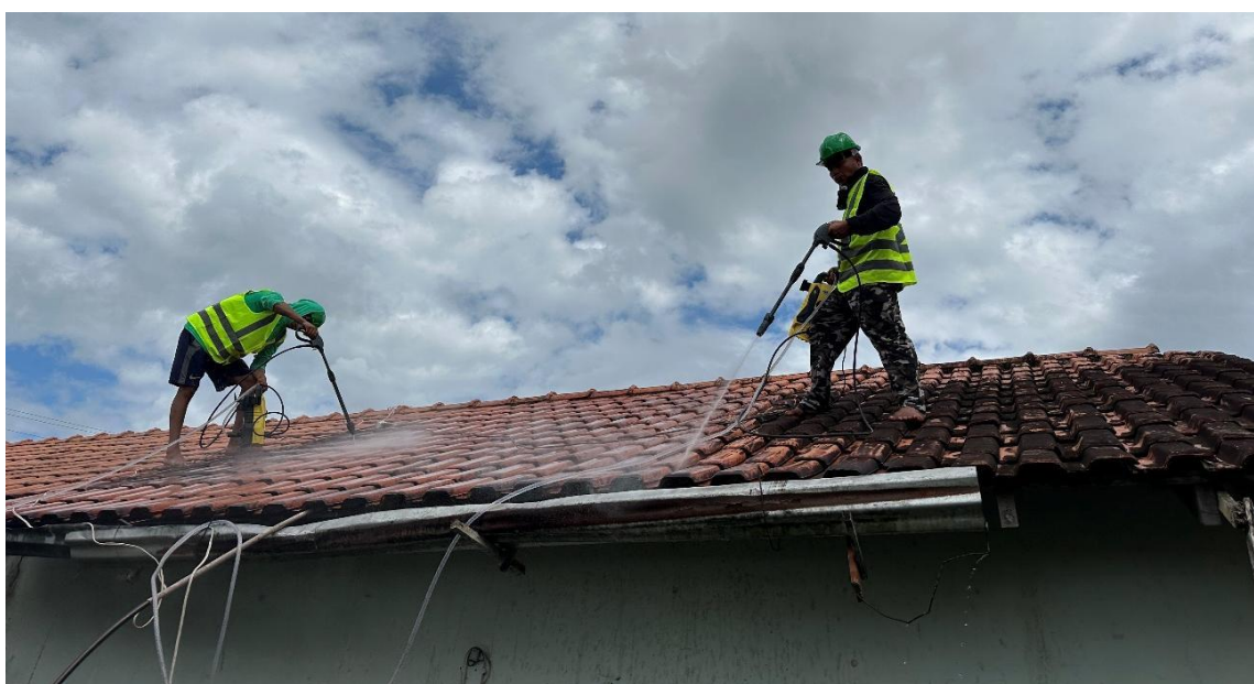
Image 1.6. Technical staff removing softened dirt with the use of pressure washers, Villa Olivença.
