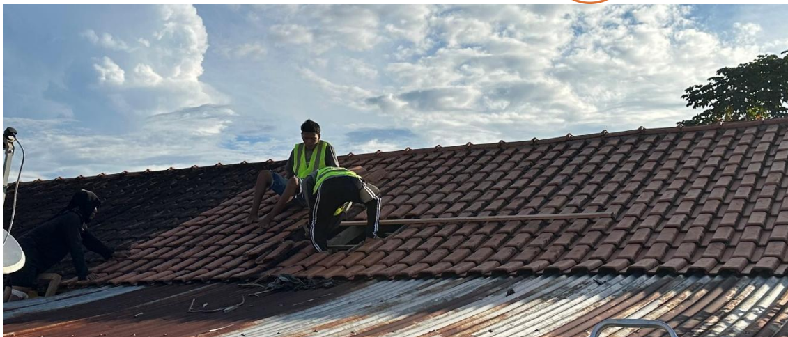
Image 1.7. Technical staff conducting the repair on the roof structure and arranging the tiles before painting, Villa Olivença.
