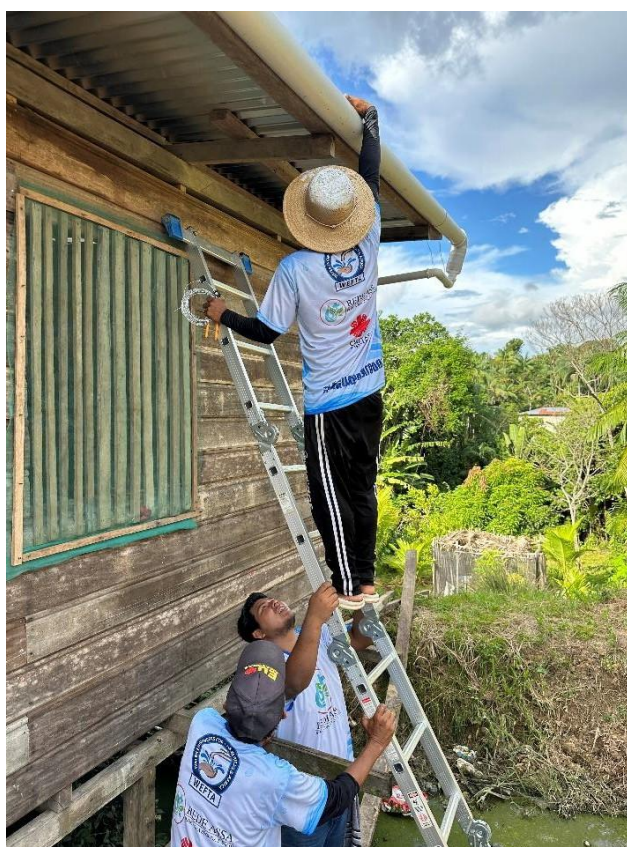
Image 1.10. Technical staff installing the gutter on the roof of a house, Villa Olivença.
