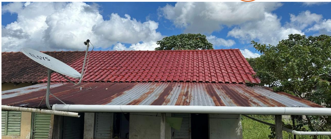
Image 1.9. View of the roof after the 2 coats of paint with liquid blanket and comparison with the roof without maintenance, Villa Olivença.
