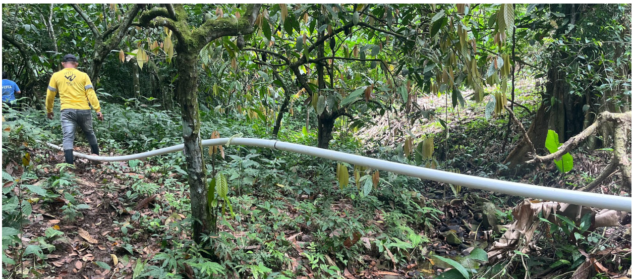
Figure 13: Mario Lopez Arriba Pipeline Bridge
