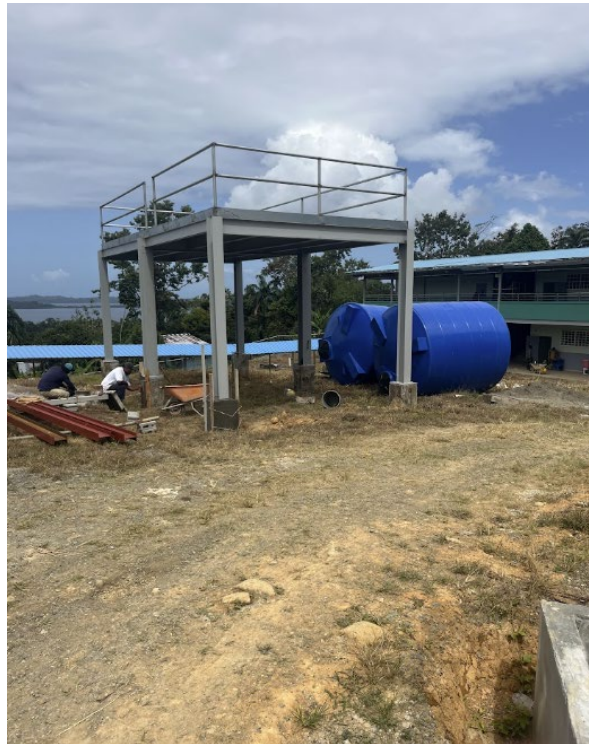
Figure 30: Proposed Platform for Storage Tanks
