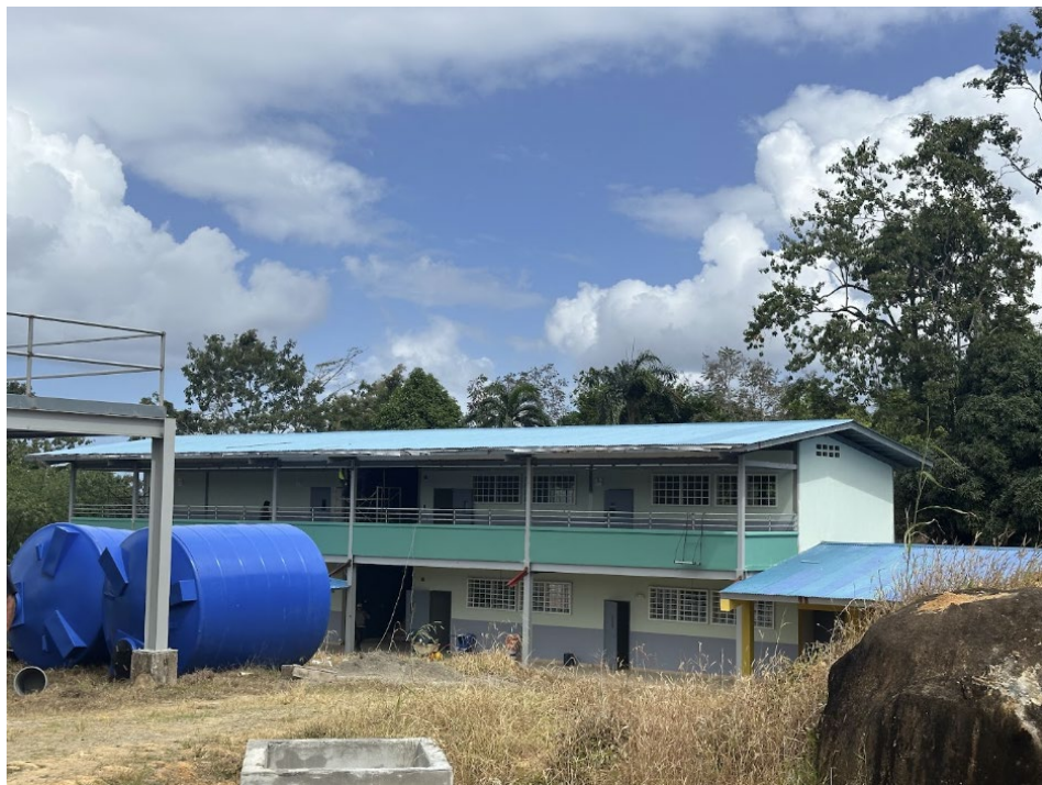
Figure 33: New High School Construction
