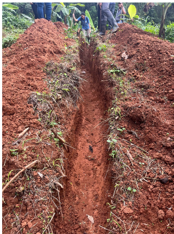
Figure 39: Rio Oeste Trench for New Proposed Pipe
