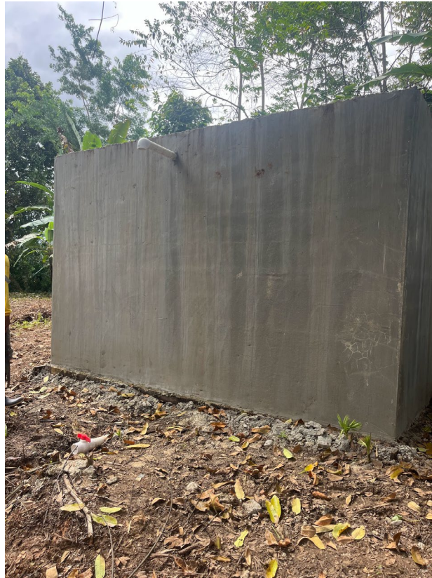
Figure 10: Mario Lopez Arriba Concrete Tank Cleanout & Overflow
