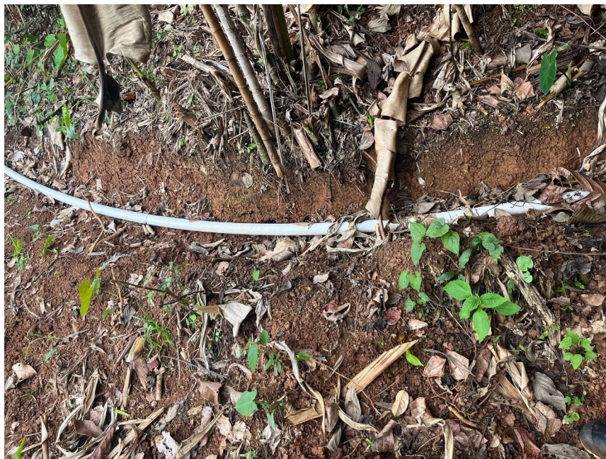
Figure 37: Rio Oeste Pipeline
