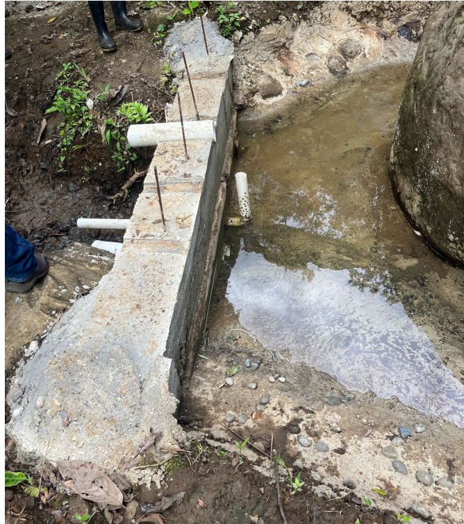
Figure 36: Rio Oeste Intake
