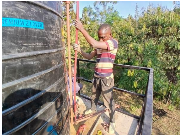
Plumbing works at the tank
