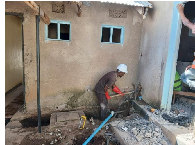
Before Renovation IPD toilet block (outside)
