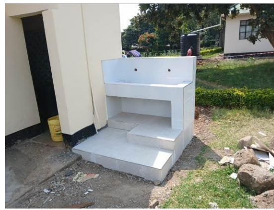
Constructed hand washing stations
