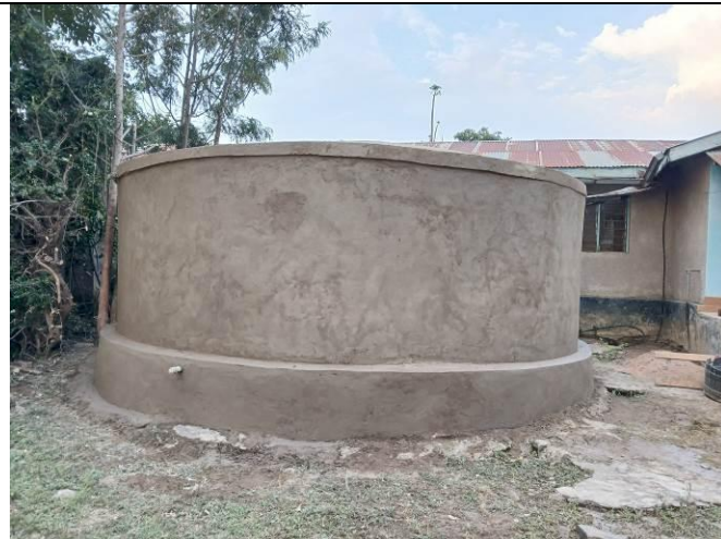
After renovation of on-ground storage tank
