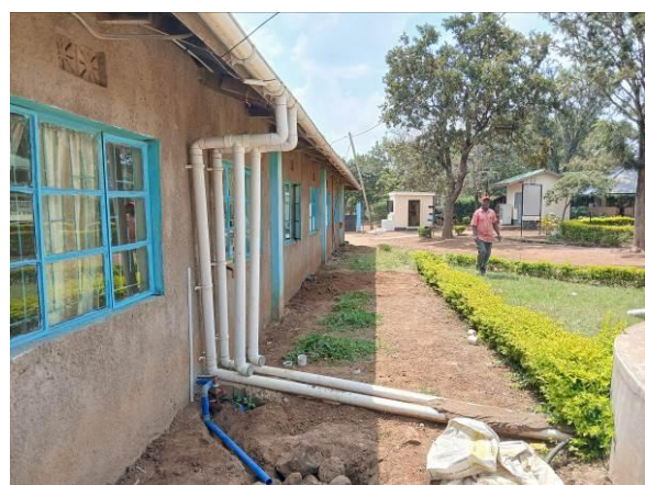
Installed first flush system
