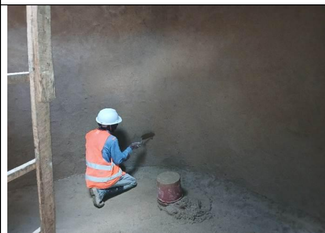
applied new plaster coat and reinforced concrete floor
