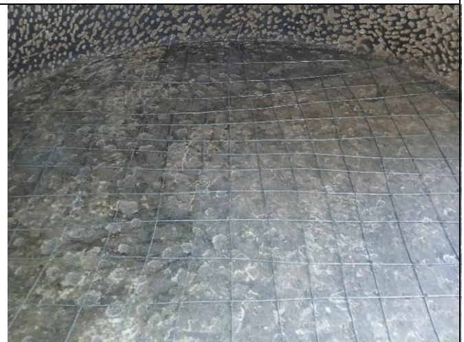
Reinforcements before concreting work
