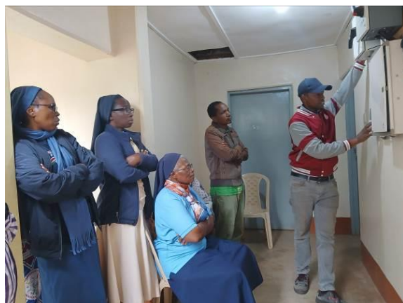
Training on the installed solar water heater
