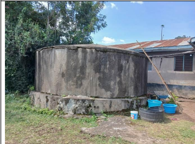
Before renovation (at the priest's house)
