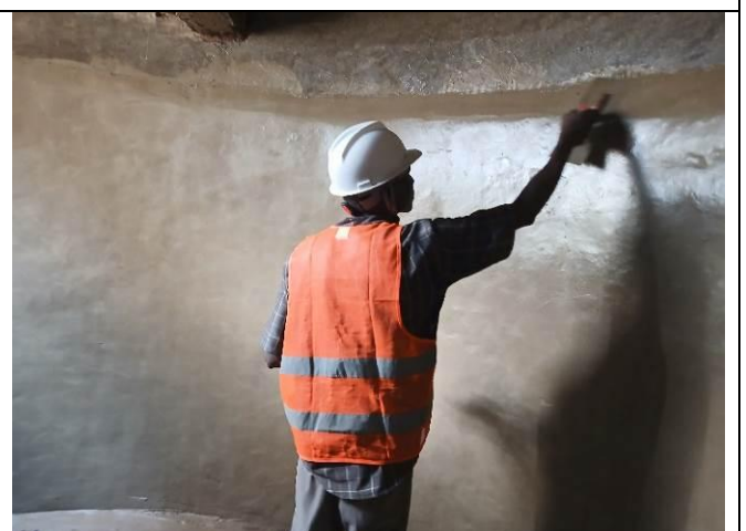
Finishing work of the applied plaster
