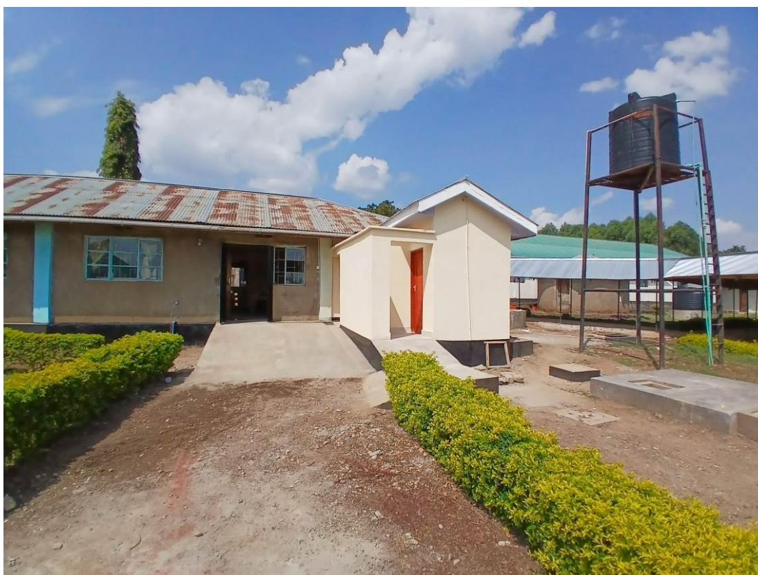
On 18 th of July 2026, Masanga health centre in Tarime DC, photo shows among of the constructed infrastructures (staff toilet block) for BMMT HC. Photo captured by Franco
