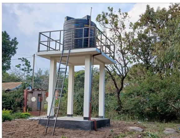
Constructed 3m tank tower
