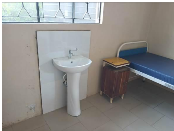
Installed wash hand basin at surgical ward
