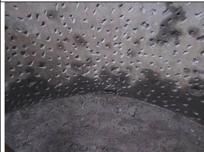
Preparation of surfaces ready replastering and floor
