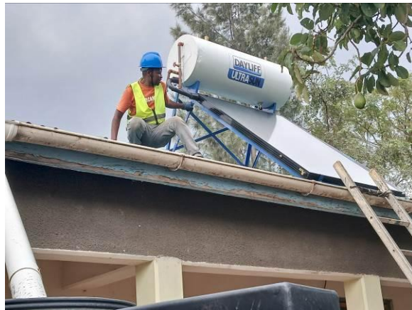
Installation of 200L solar water heater
