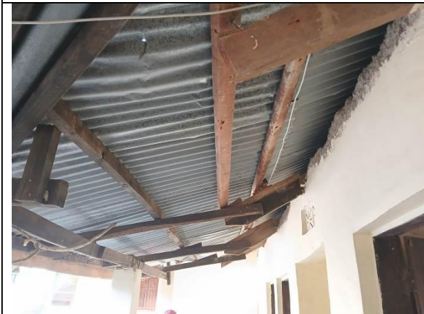
Before renovation of IPD toilet block's corridor
